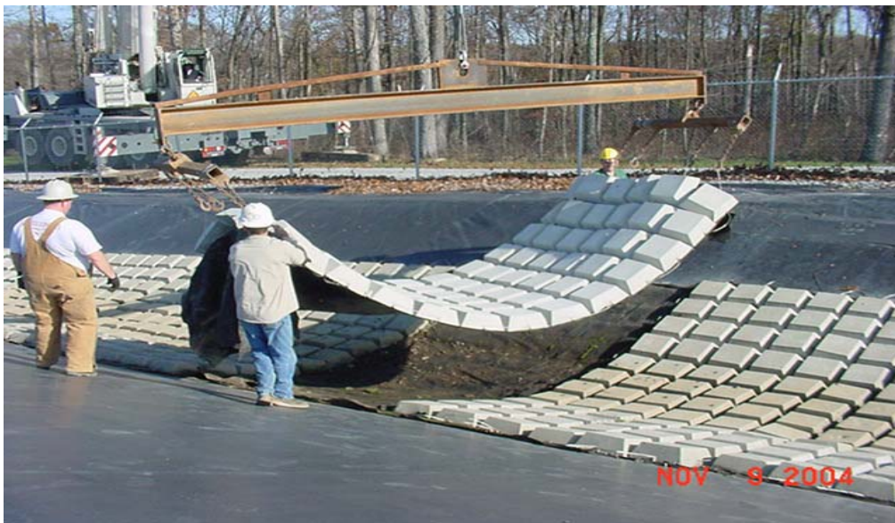
Photo 3 New cc45 mat being installed Photo by T. Stewart
