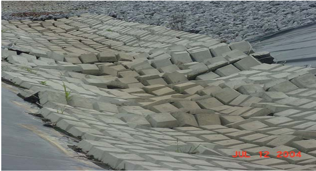
Photo 1 AB mats in South Channel following major rain event. Photo by Jeff Stamper.
