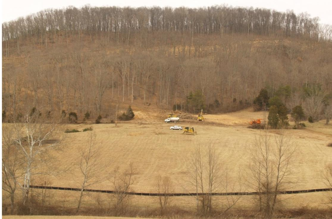
*The haul road, seen on the hillside, is being cut from the borrow area in the valley up to MFDS. The field seen in the foreground is the primary borrow source and it will feature a storm water detention pond. Silt fences are being installed adjacent to all excavation sites to protect Rock Lick Creek.*
