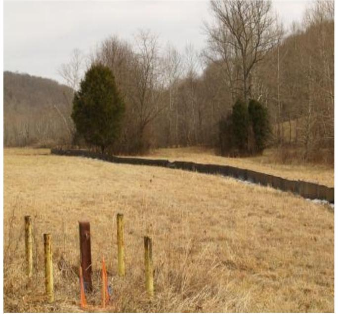
*This silt fence was installed adjacent to the protective riparian area of Rock Lick Creek to reduce runoff from the primary borrow area and protect the creek.*
