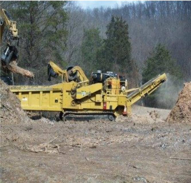
*Cleared timber and brush are being chipped on site and will be recycled and used in erosion control measures.*
