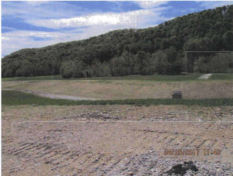
99. SWMF #2 located at the base of the hill on the east side of the LF.
