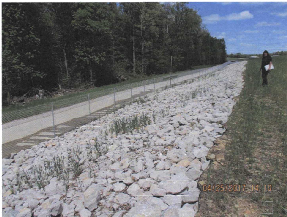
167. Stone and drainage on the west side of the LF.
