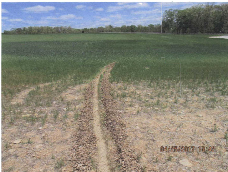
148. Wood chips from erosion control sock remaining on the LF after removal of the outer fabric, located near the East Basin.
