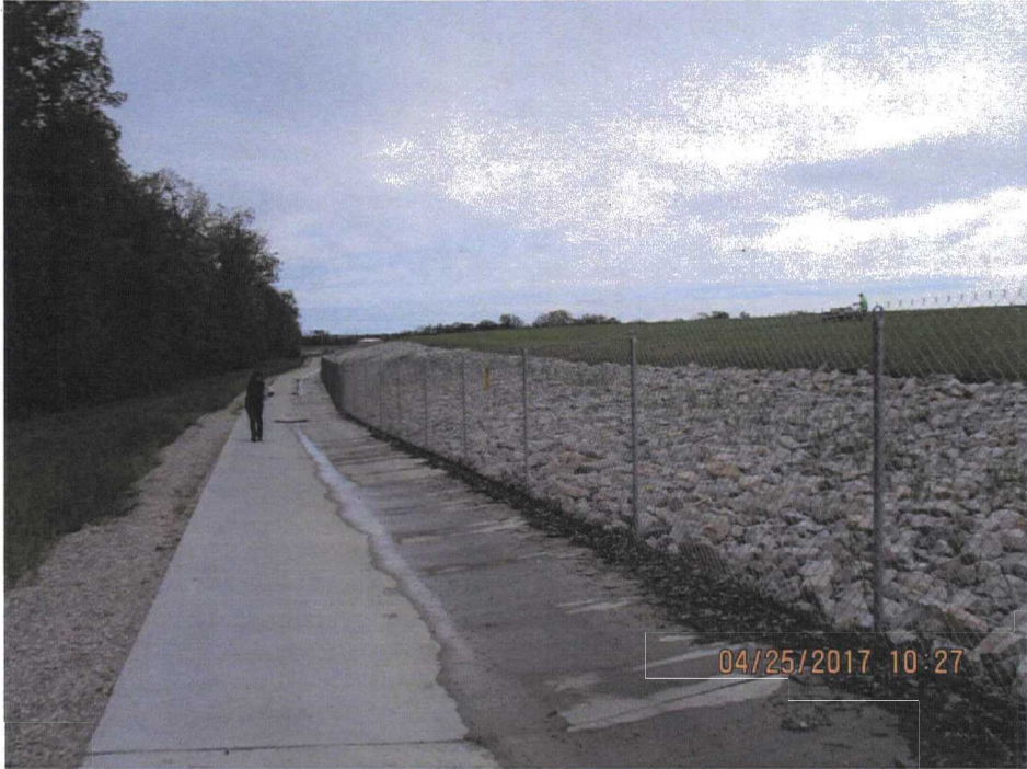
19. West side of the perimeter road.
