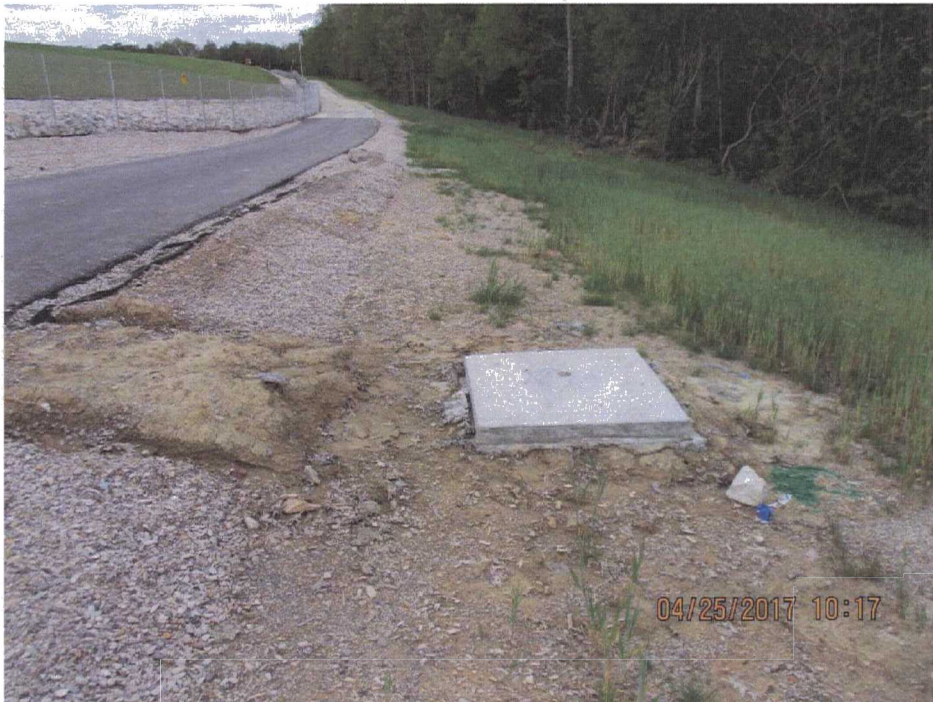
8. Survey monument near the northwest corner of the LF.
