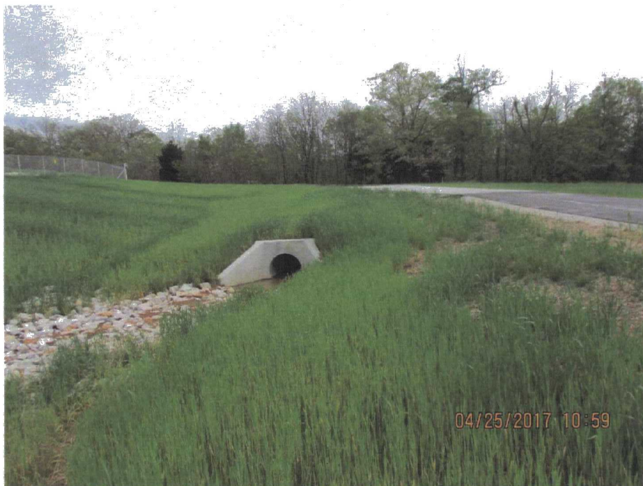
66. Storm drain outlet near the northeastern corner of LF.
