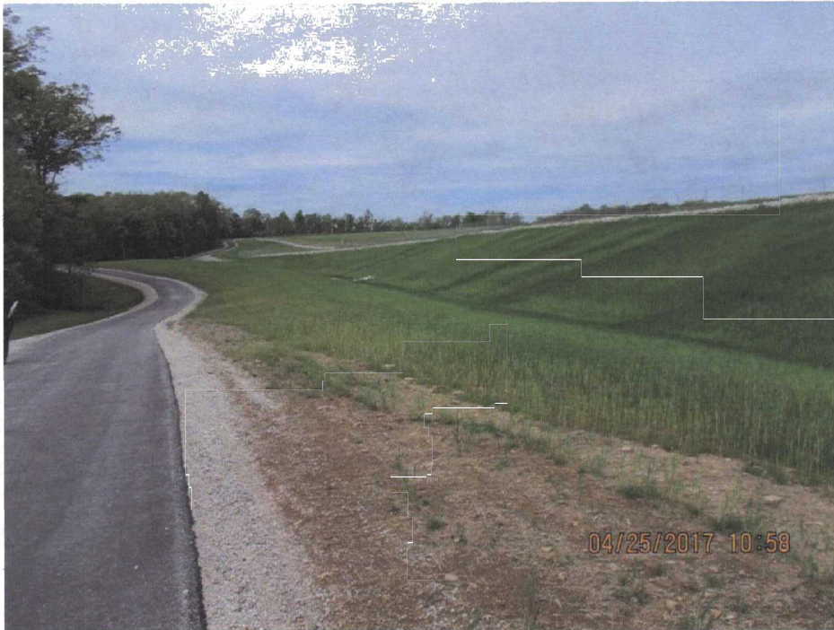
65. East perimeter drainage.
