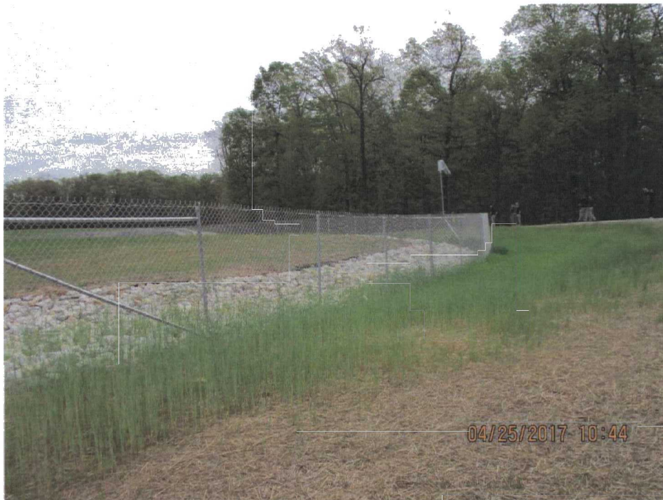
42. Southeast corner of the LF.
