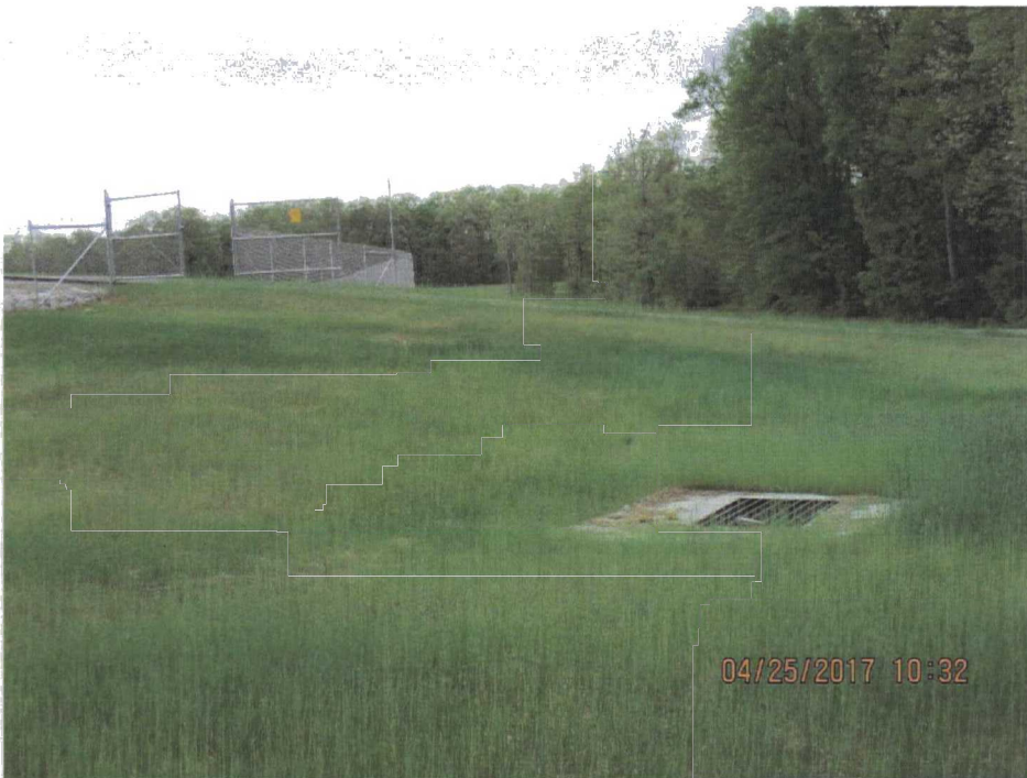
24. Southwest corner fence with access gate and storm drain.
