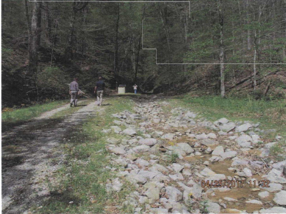
93. East drainage at the base of the hill.
