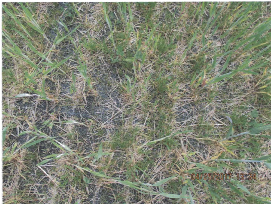
142. Close up of an area with TRM that drains towards East Basin.
