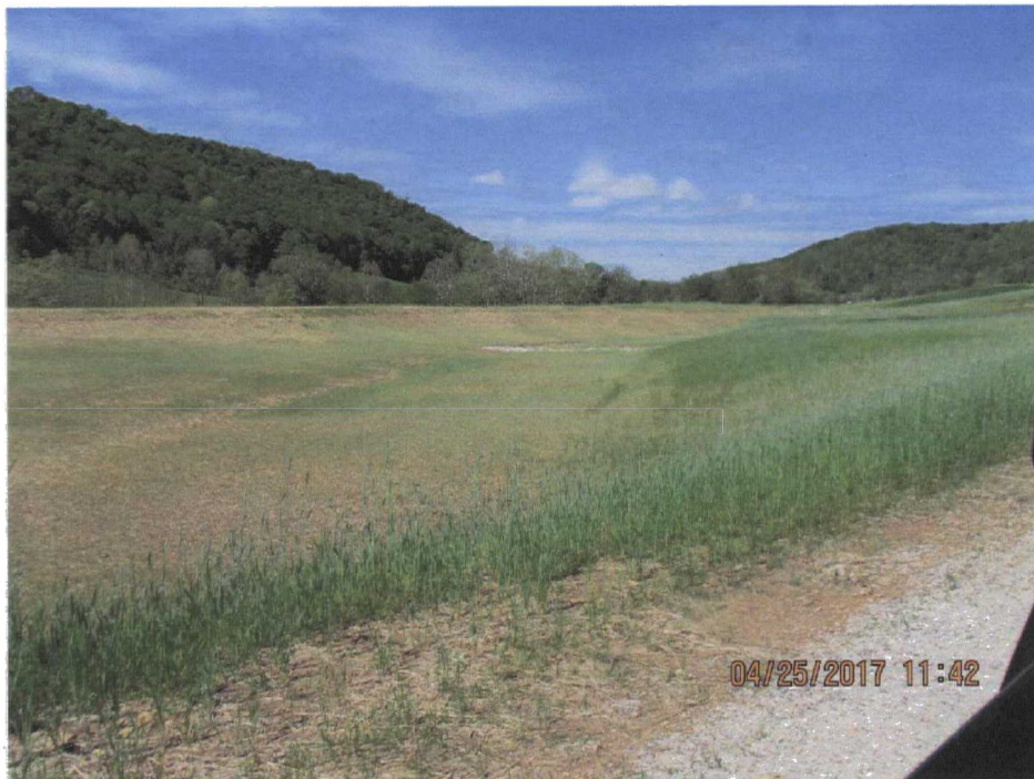
98. Surface Water Management Feature (SWMF) #2 located at the base of the hill on the east side of the LF.
