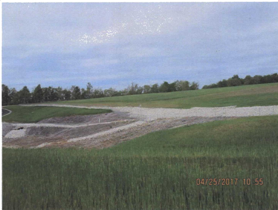
62. Fence between LF cap and the East drainage basin at the LF east perimeter.
