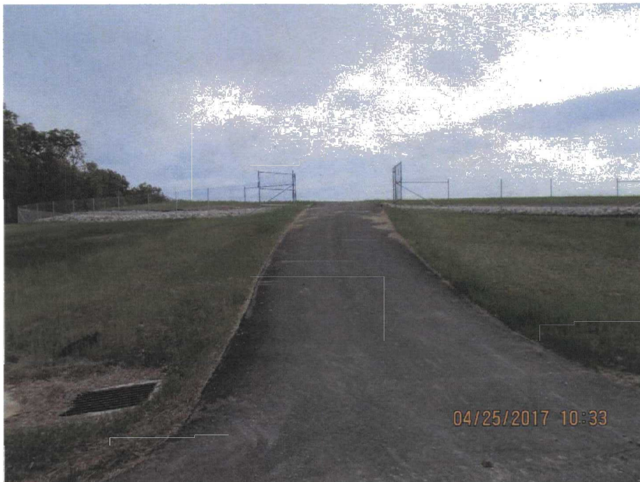
26. Access gate at southwest corner of the LF.
