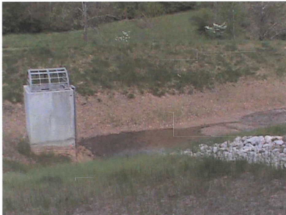
106. Close up of SWMF #3
