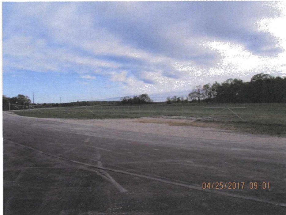
2. Former borrow area at the entrance to site.
