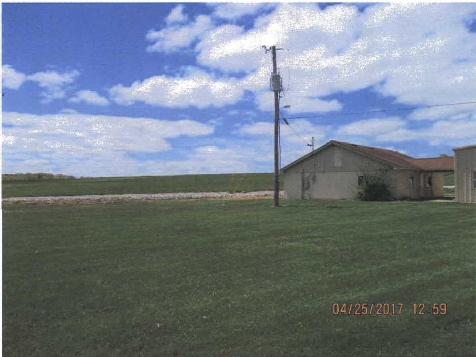
116. The north side of LF with the KyDEP office visible on the right.
