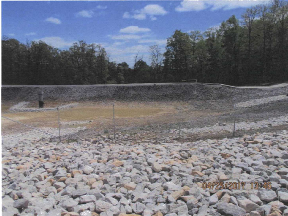
153. Panorama of east drainage basin from south to north (Photo 2 of 4).
