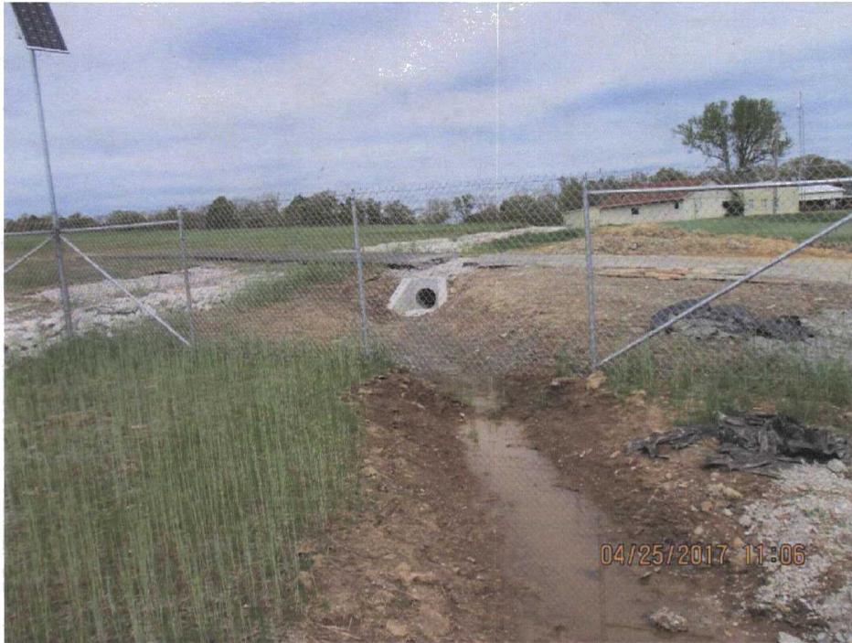
75. Storm drain at the northern perimeter under the access road to the LF cap.
