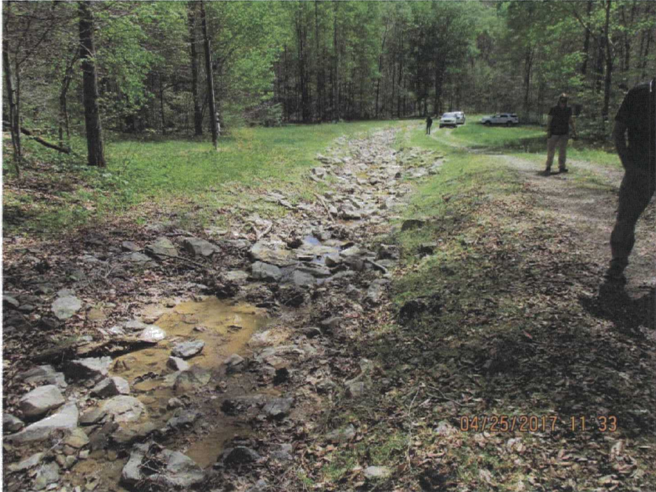
95. East drainage at the base of the hill.
