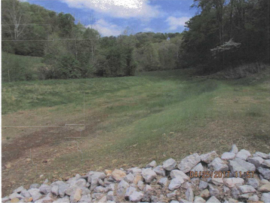
107. The northern portion of SWMF #3.
