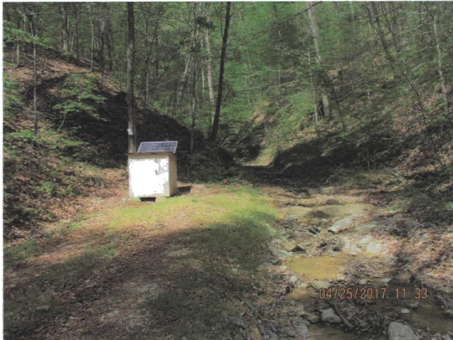
94. East drainage at the base of the hill.
