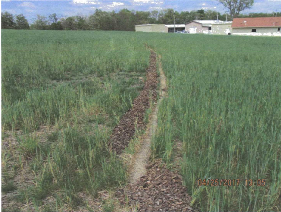
119. Wood chips from an erosion control sock remaining after outer fabric was removed.
