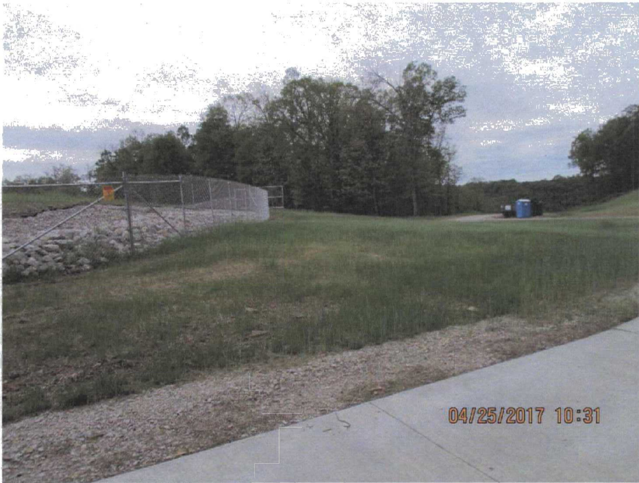
23. Southwest corner of LF cap and the haul road leading to borrow areas over the hill to the right.
