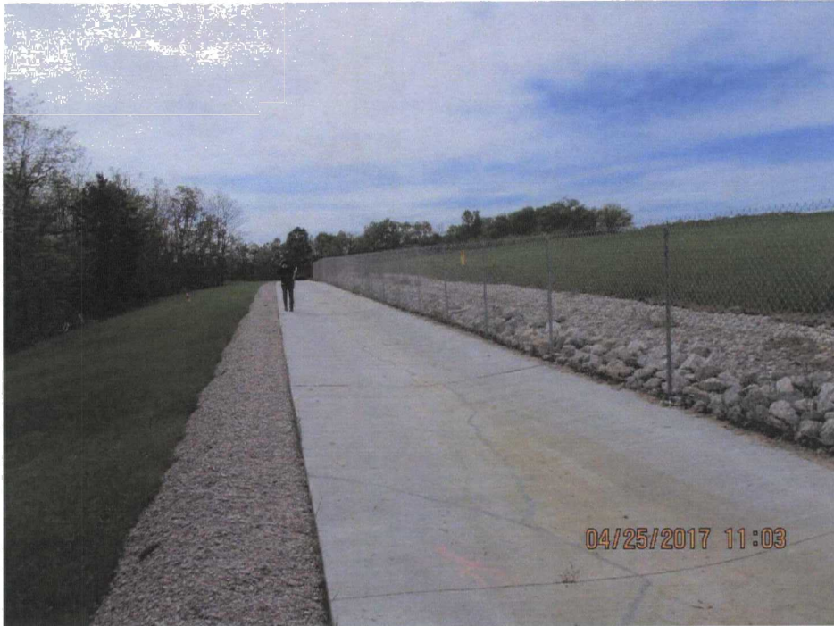
73. Northeastern perimeter road and drainage.
