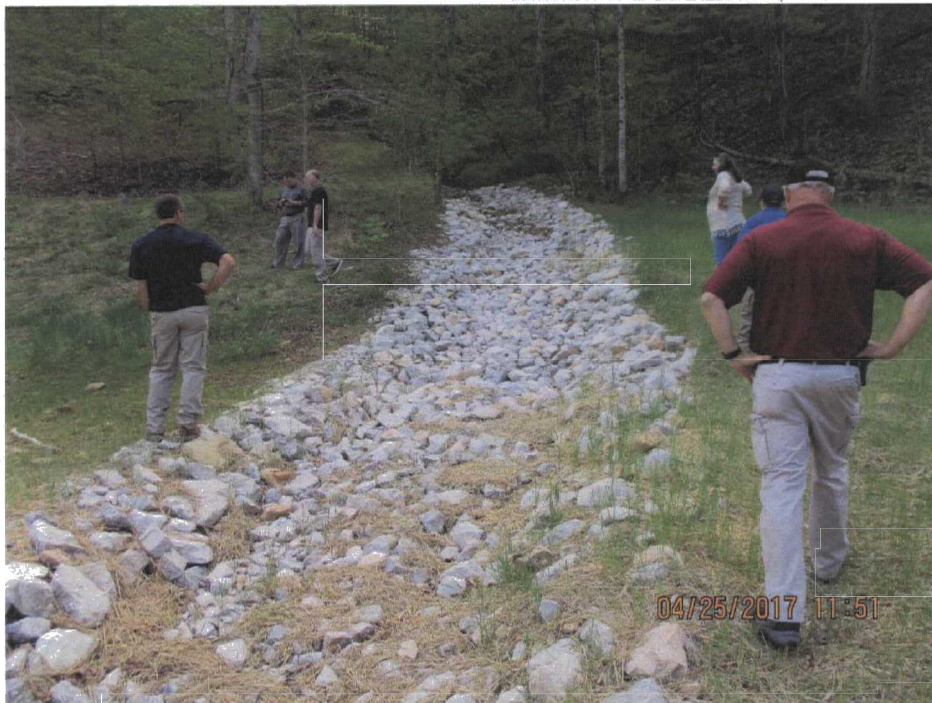
101. Drainage path into SWMF #3.
