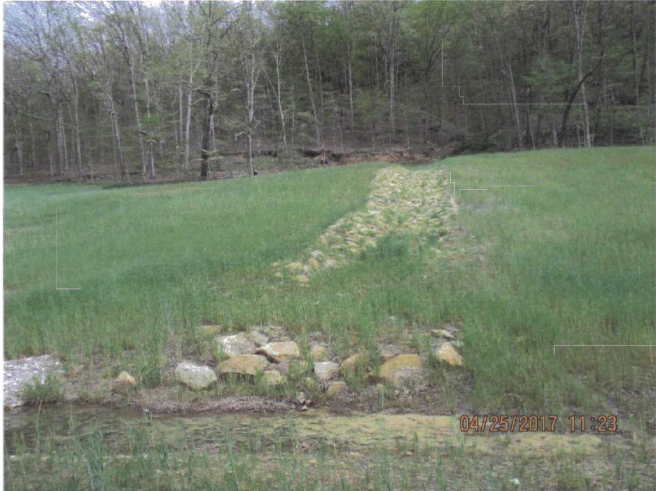
84. A slip on the hillside and constructed drainage in the former Borrow Area #4.
