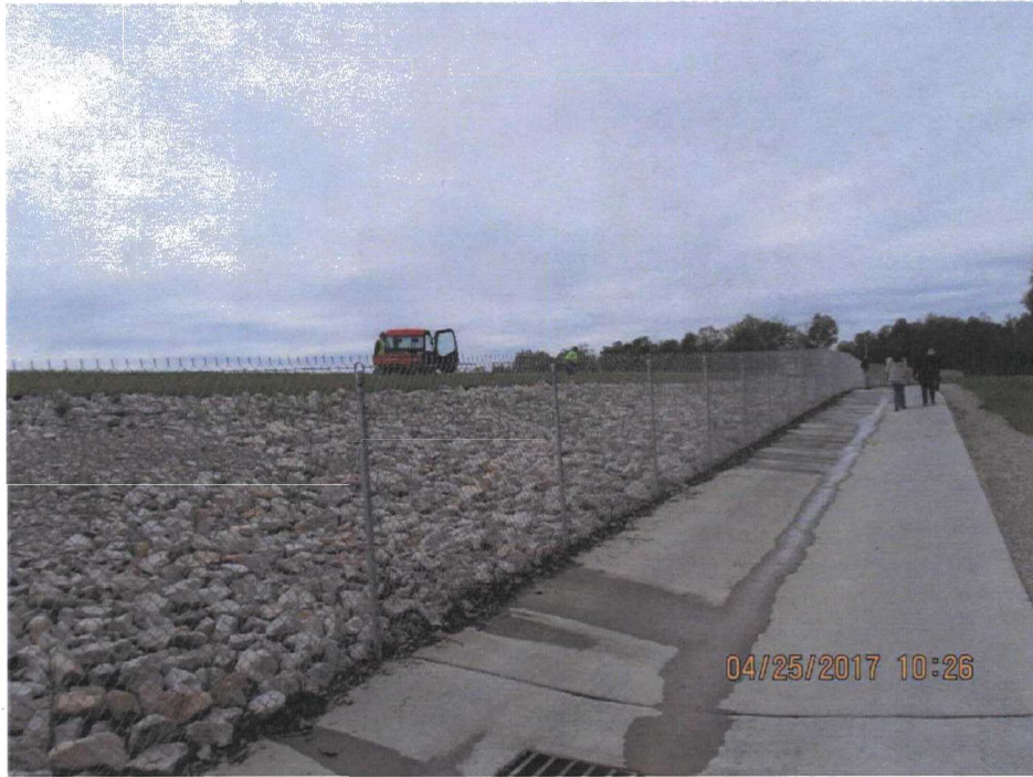
17. Contractors picking up rocks on the LF cap.
