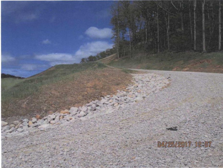
113. The haul road taken from bottom of hill.
