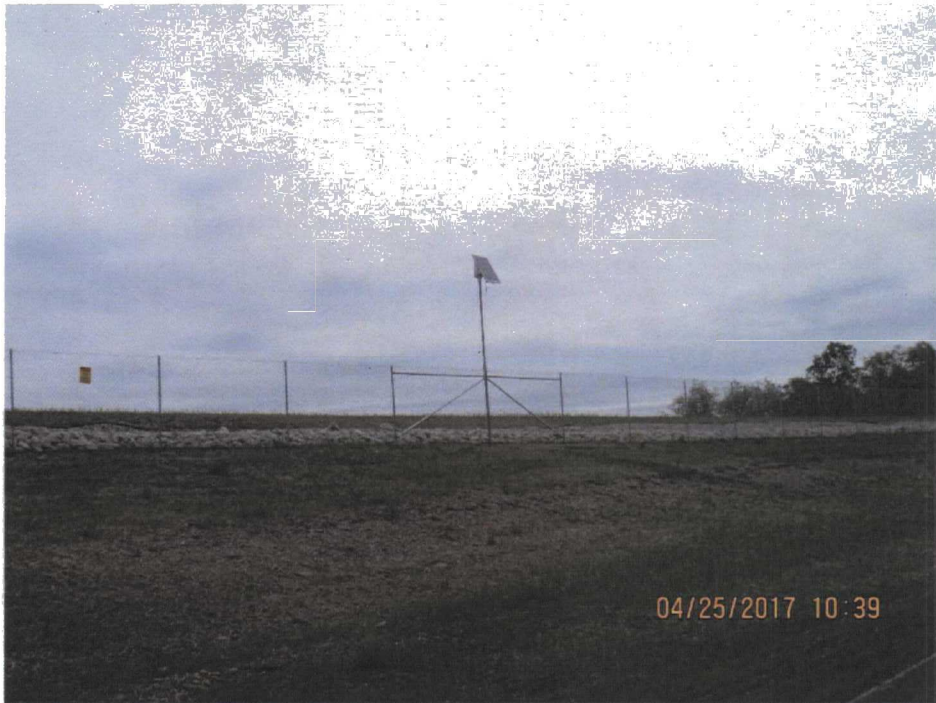
36. Solar panels to power perimeter lighting.
