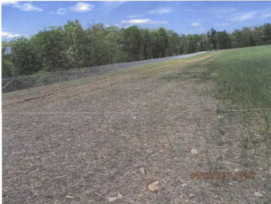
161. Sparse vegetation near the southern end of the LF near the fence.
