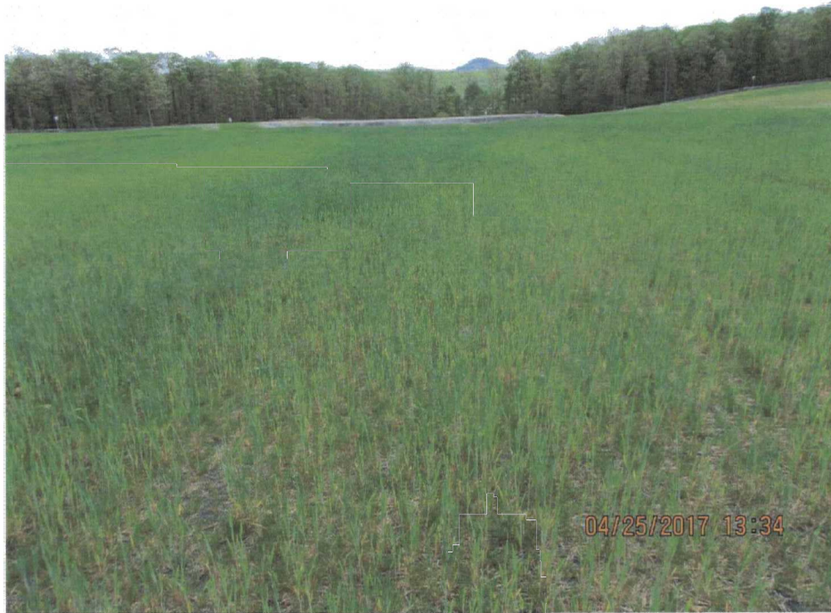
141. An area with turf reinforcement mat (TRM) that drains towards East Basin.
