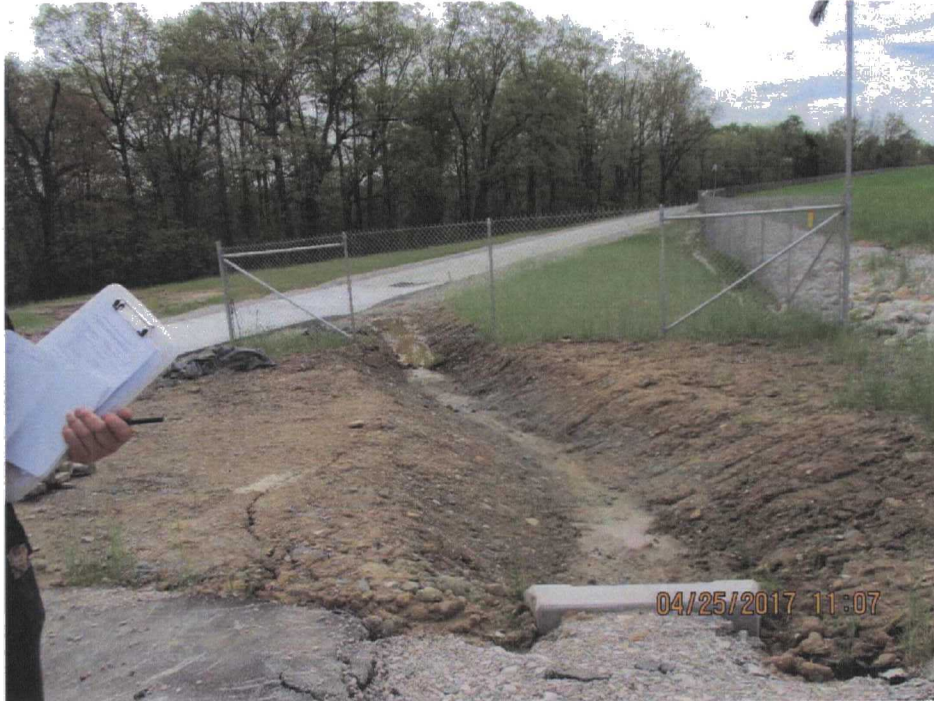
77. Drainage and access gate at the north end of the LF.
