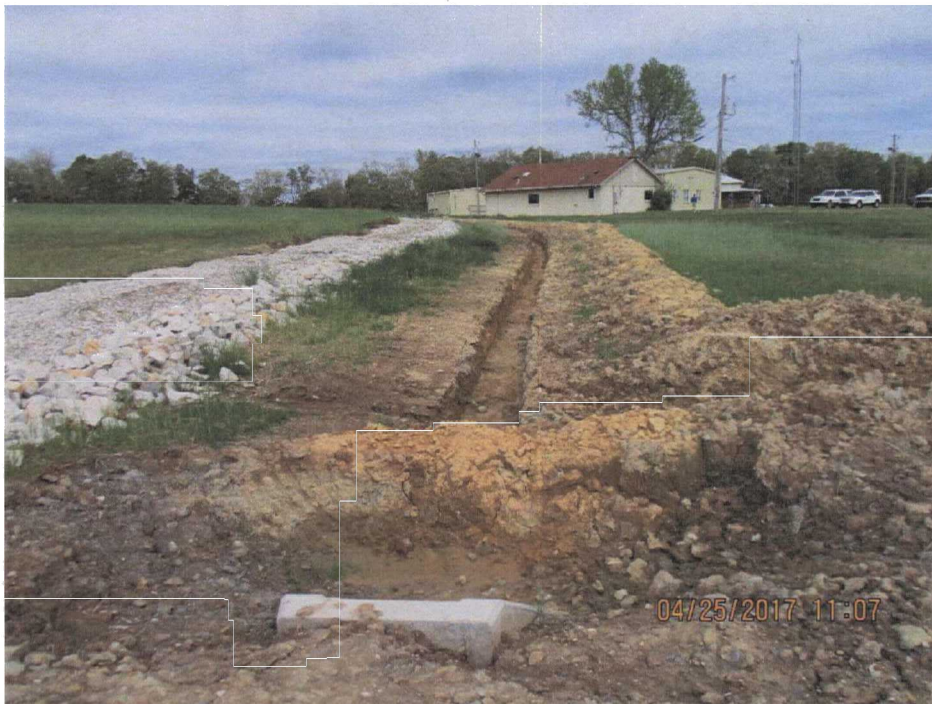
76. Drainage construction along the northern perimeter of the LF.
