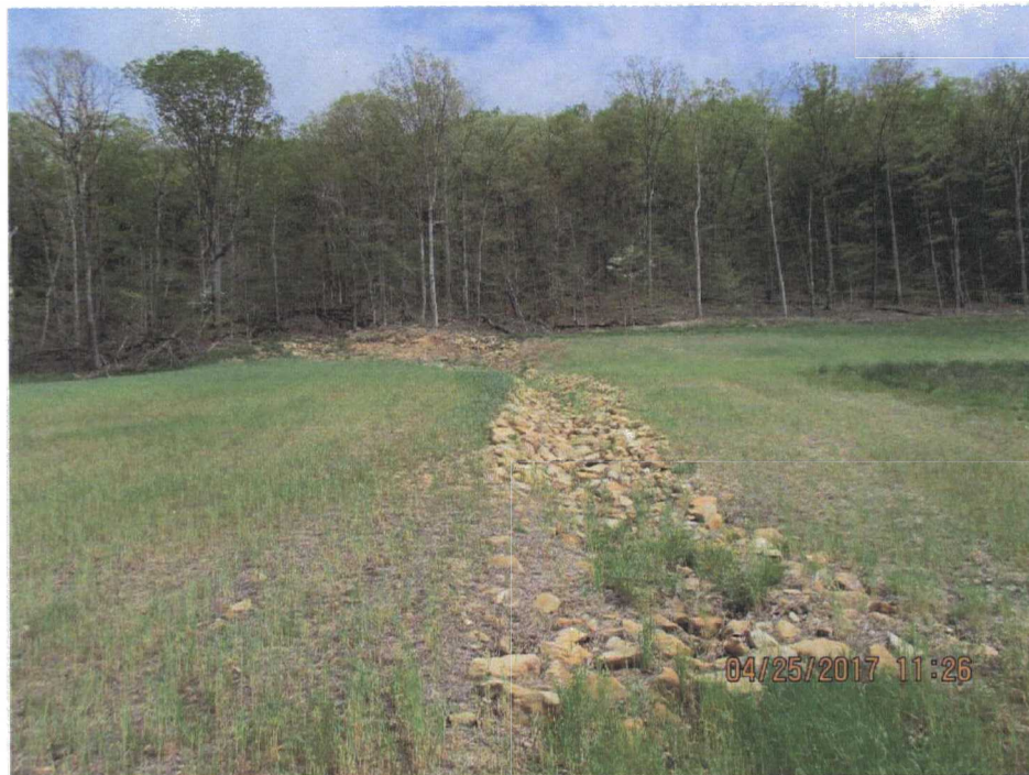
90. Constructed surface drainage in slip area, Borrow Area #4.
