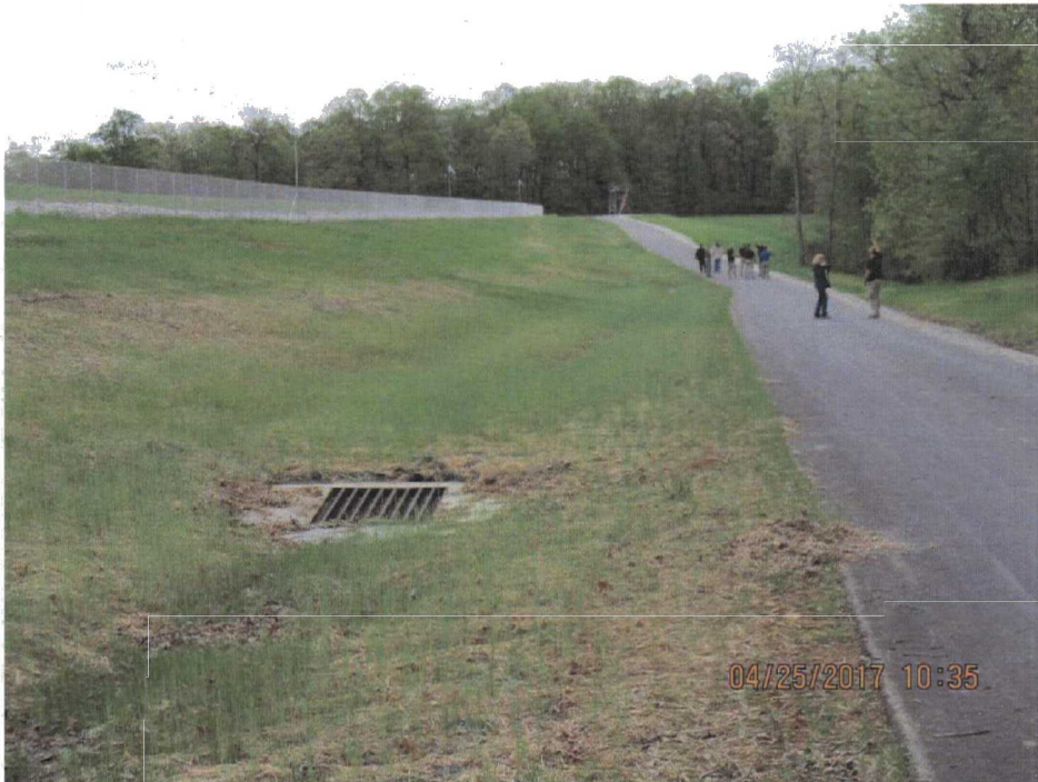
28. Storm drain along the south perimeter road.
