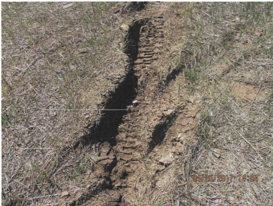
164. Close up of tire ruts in the LF cap near the southwestern access gate.
