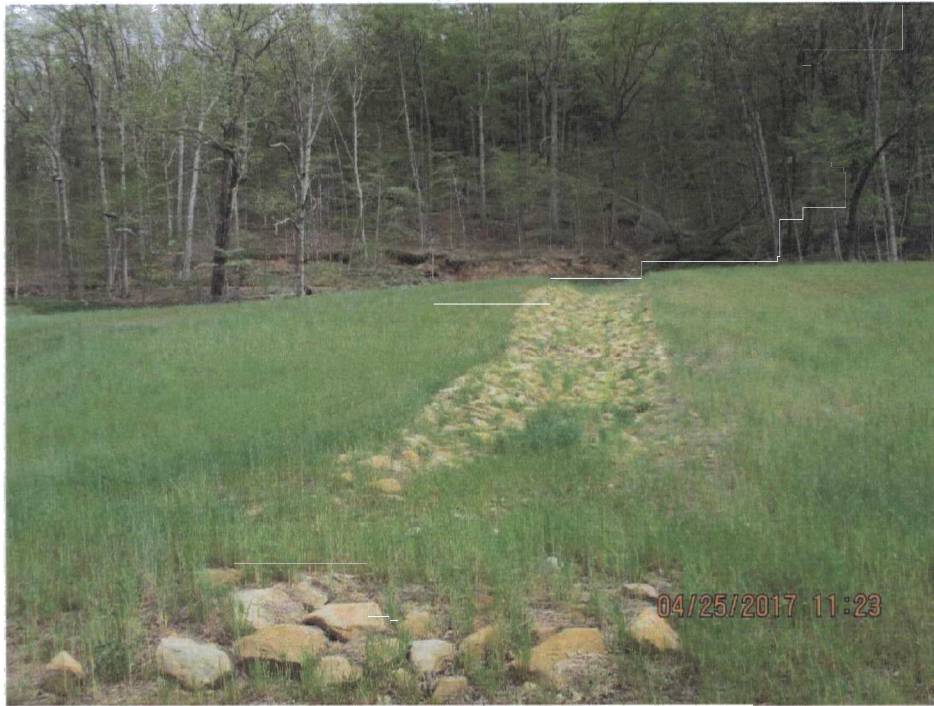
85. A slip on the hillside and constructed drainage in the former Borrow Area #4.
