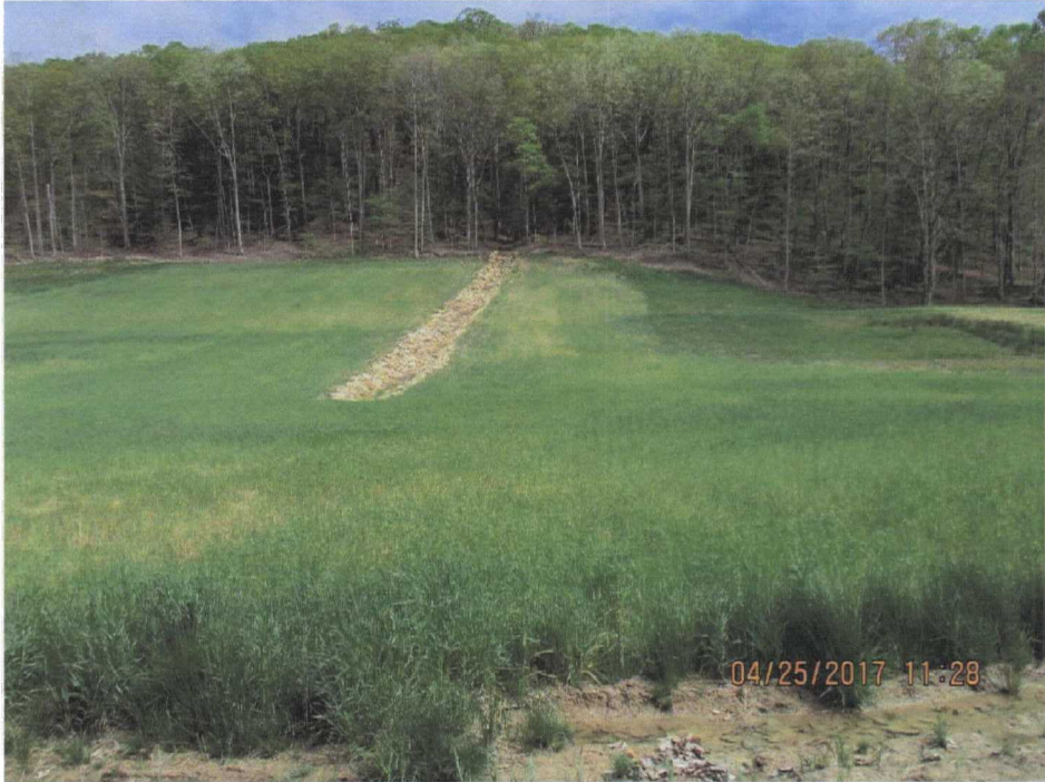
91. A surface drain constructed on the hillside in Borrow Area #4.
