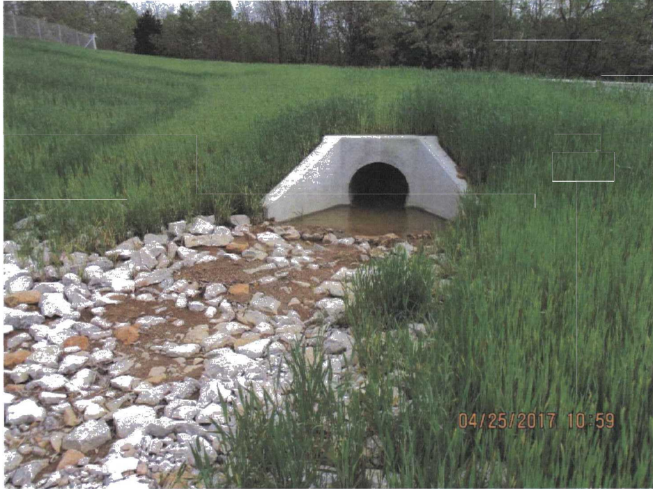
67. Close up of a storm outlet near the northeastern corner of the LF.
