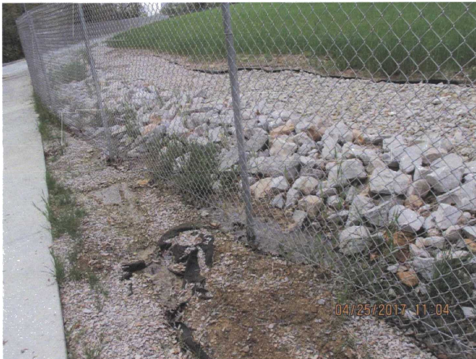
74. Water drainage along the edge of riprap at the edge of the LF.
