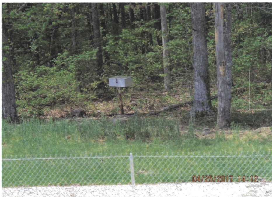
168. A monitoring well to the west of the LF.
