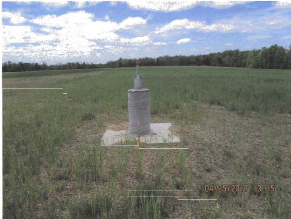
130. Mount for a closed-circuit television (CCTV) surveillance system on top of the LF cap.
