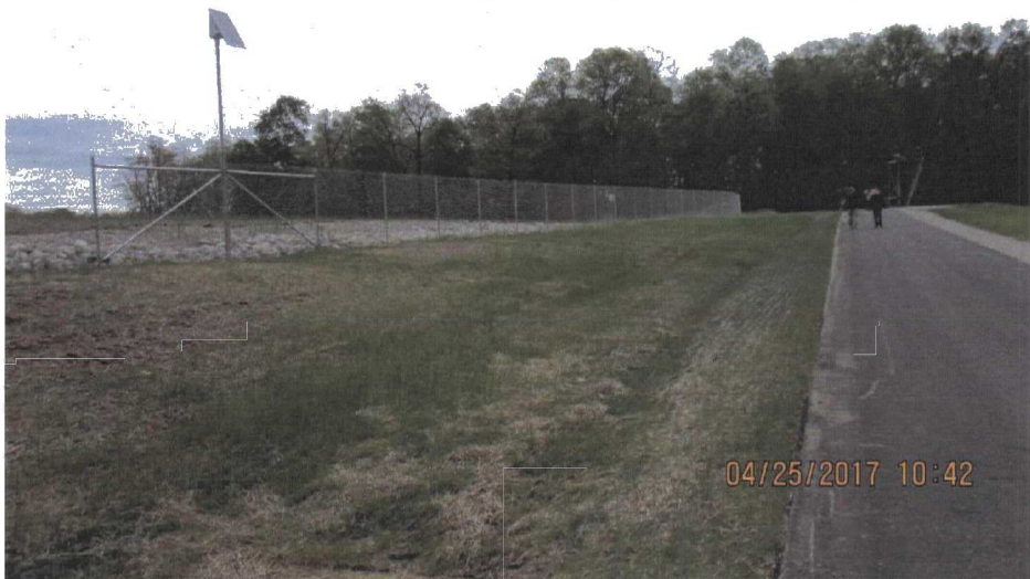
40. Solar panels near southeast corner of the LF.
