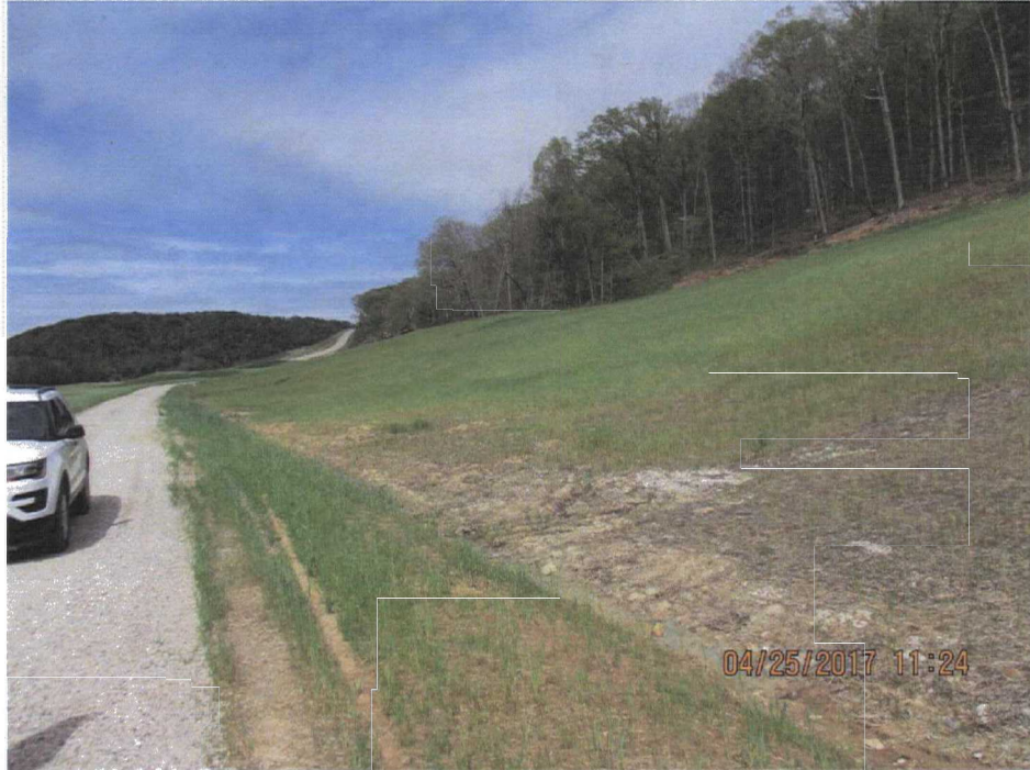
87. Hillside where slip occurred in Borrow Area #4.
