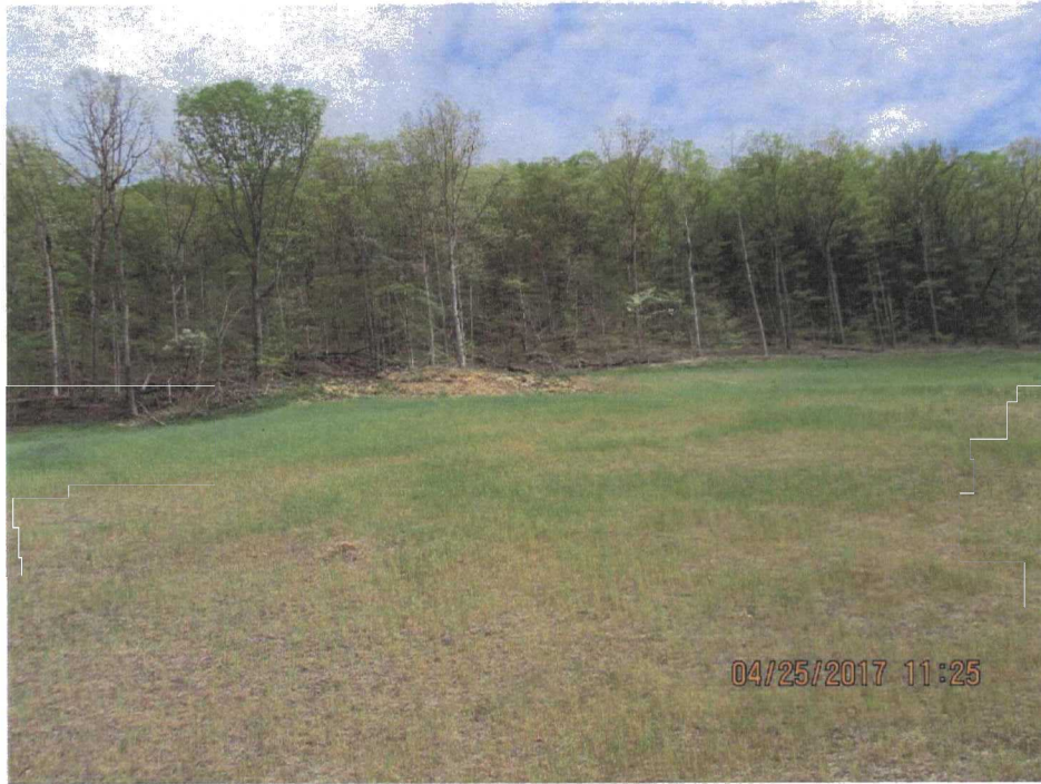
89. Hillside where slip occurred in Borrow Area #4.
