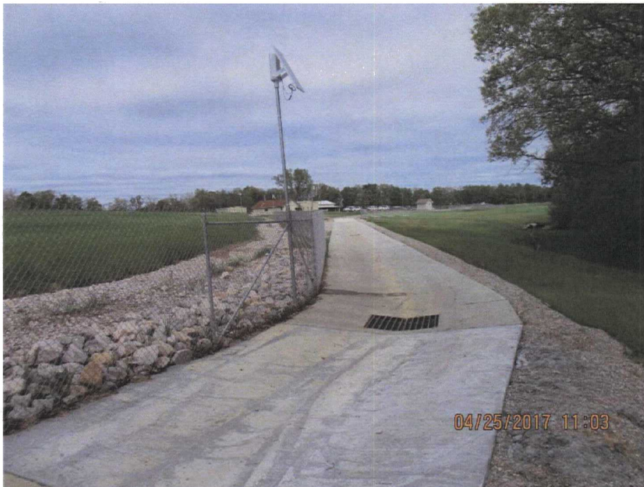
72. LF fence and storm drain in the northern perimeter road.
