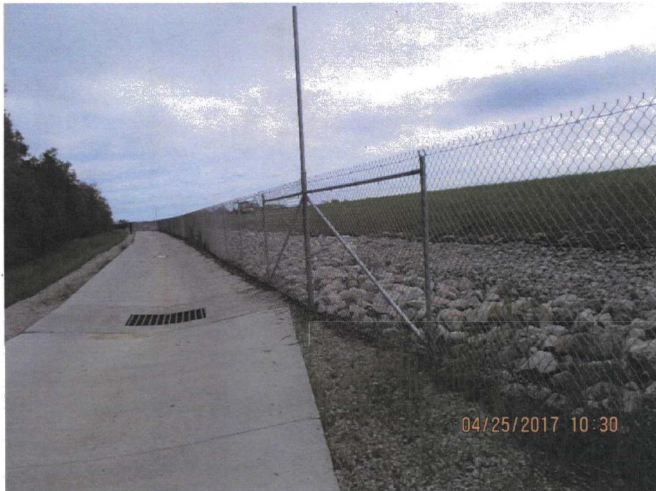
22. West perimeter road and fence.
