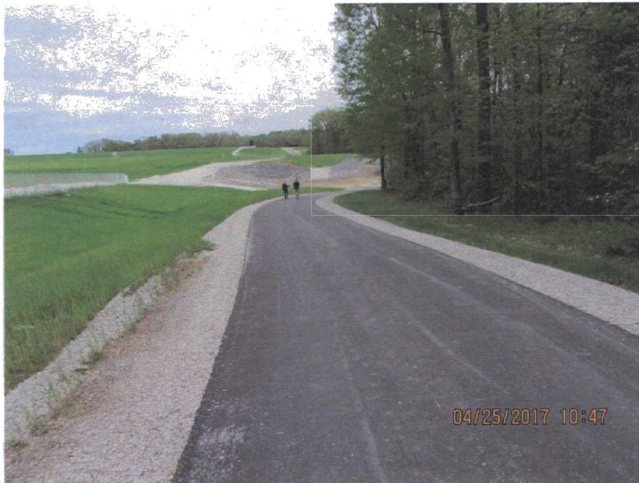
50. The east perimeter road and east drainage basin in the distance.
