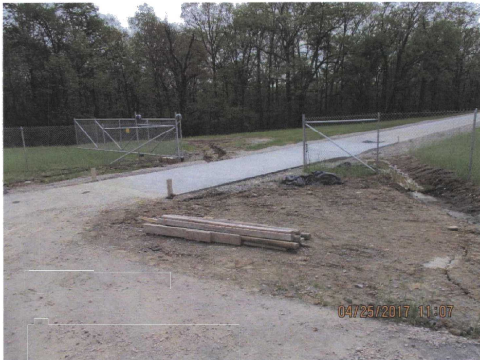
78. Drainage and access gate at the north end of the LF.
