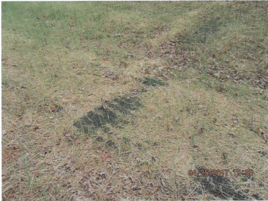
29. Turf reinforcement mat in drainage path near the south perimeter road.
