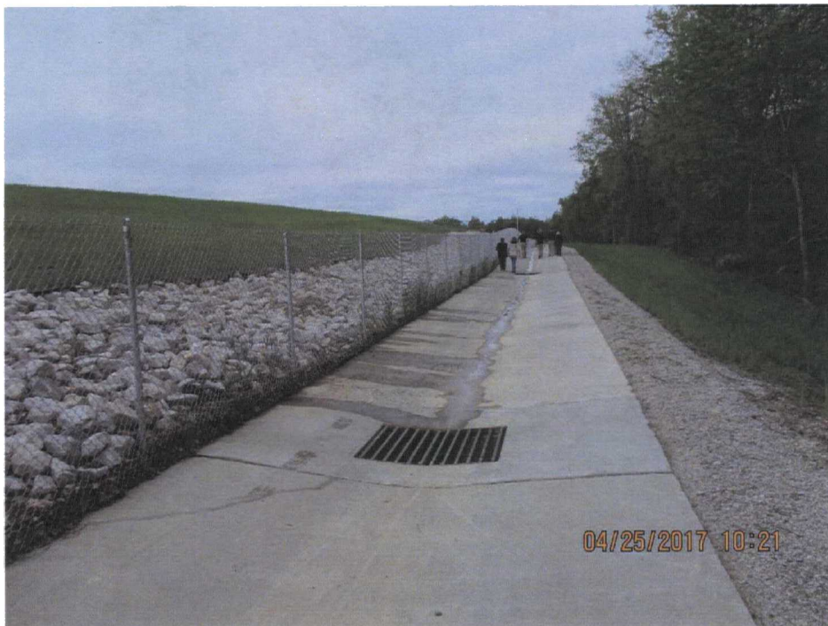
14. West side of the perimeter road.
