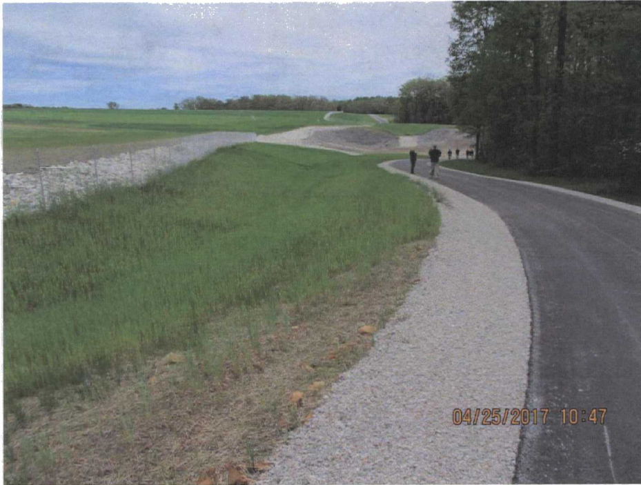
49. Drainage path between the LF cap and the east perimeter road near the southeastern corner of the LF.
