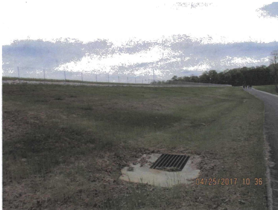
30. Drainage along the south perimeter road.
