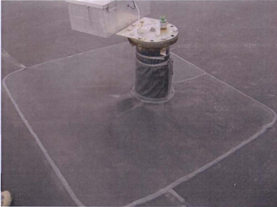
Photo 3: Typical Sump with Liner Boot
