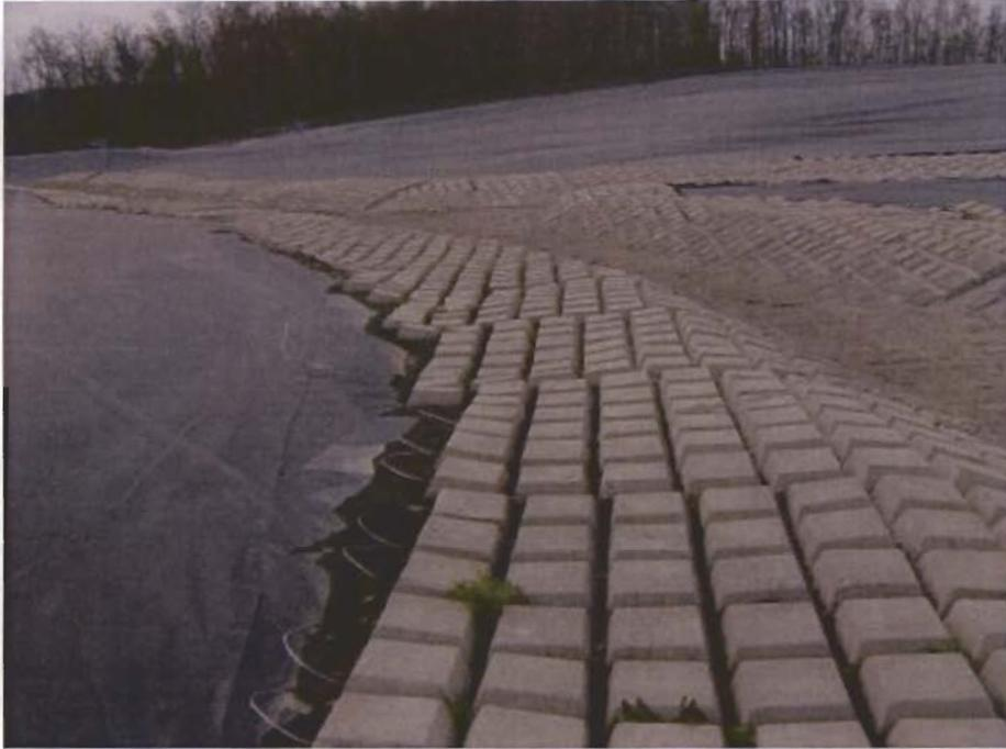
Photo 9: Y-Channel Revetment
