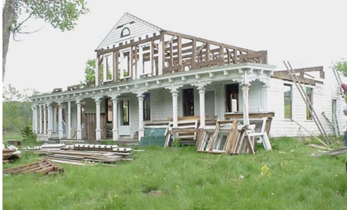
Dismantling of Bruchmann residence, May 2000
