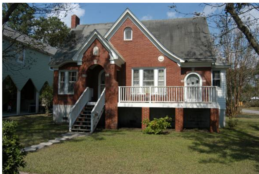
Frame building elevated on concrete block foundation faced with brick veneer. Belhaven, North Carolina.
