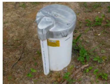
Properly tagged water well. Photo by DOW staff
