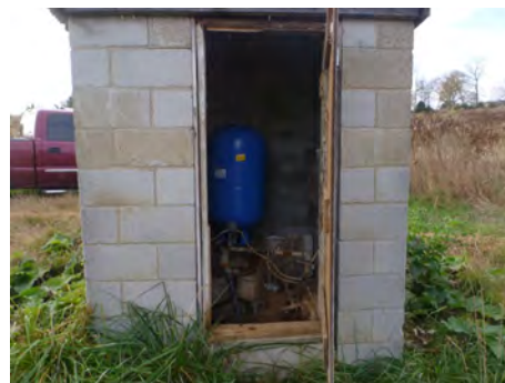
Open well house with well, piping and pressure tank. Photo by DOW staff.
