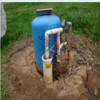
Private water well and pressure tank. Photo by DOW staff
