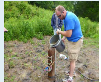
Amos Moses pouring bleach down water well. Photo by DOW staff
