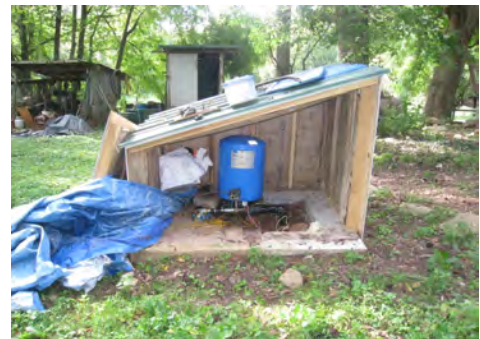
Open well house with well, piping and pressure tank. Photo by DOW staff.
