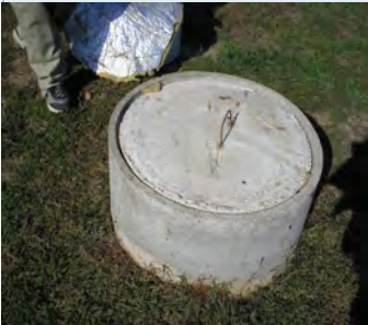
Tile casing and concrete lid private water well. Photo by DOW staff.
