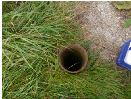
Open well with steel casing. Photo by DOW staff.
