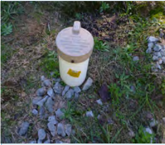
Well casing and well cap for private water well. Photo by DOW staff.
