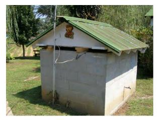
14. If the wellhead is buried or in a pit it should be brought into compliance with current regulations by a certified water well driller, the wellhead should be brought above ground level.
