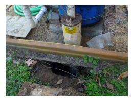
2. Well cap (cap on top of casing) Check the condition of the cap and any seals present. Insure that it is securely attached, and that it will keep out insects and rodents. If not, contact a Kentucky certified water well driller for assistance to repair it.
