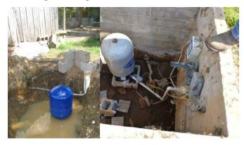
15. If your well is located in a low-lying area prone to flooding, you should consider having your certified water well driller raise the well casing to at least 24 inches above the historic record flood level, properly sealing the wiring conduit and providing casing bumper protection if floating debris is a concern. Another option is to construct a new well at a location outside the flood-prone area.
