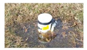
16. The well should not be in a roadway or driveway. If the well is within close proximity to a roadway or driveway, it should be properly marked to avoid being hit by vehicles. You can protect your well by placing bumper posts near the well's vulnerable position(s) to increase visibility.
