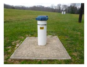
3. A certified water well driller can evaluate other considerations for the condition of the well. A compromised wellhead (cap) may allow an entry way for ants, bees, spiders, field mice, earwigs or other critters into the well and water supply.
