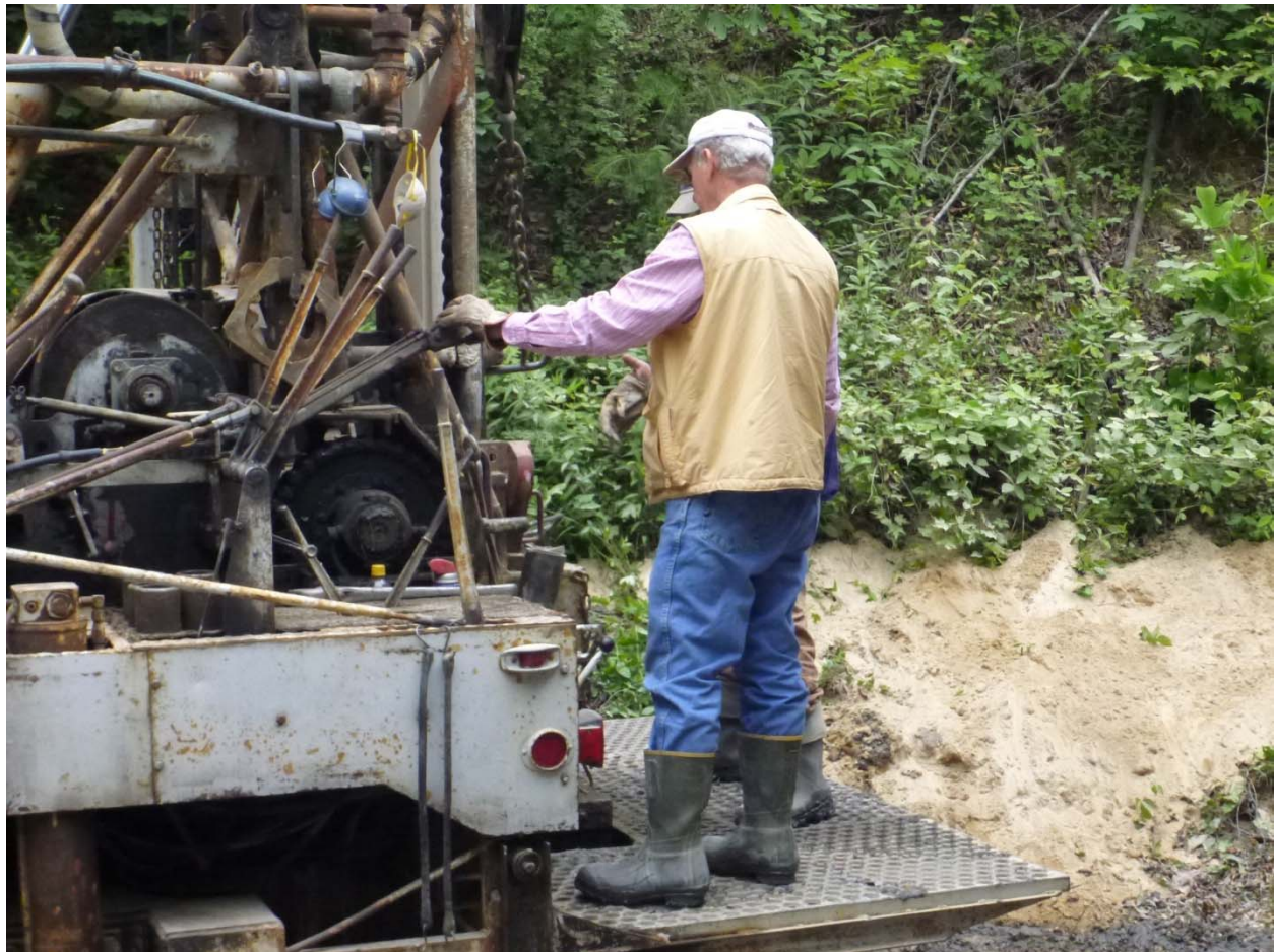
Certified Water Well Driller Billy Lewis and helper of Lewis Water Works, drilling a water well in Lee County Ky. By groundwater staff.
