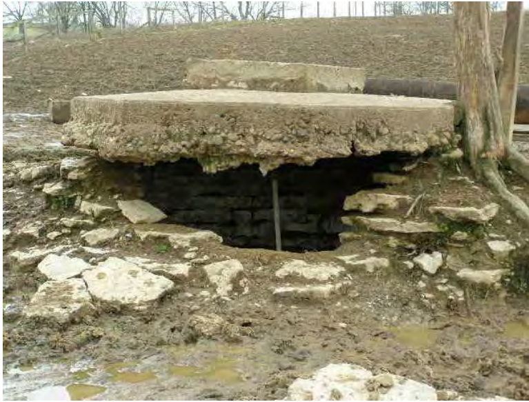
Figure 1. This abandoned well has an open side, which makes it possible for pollutants to enter the aquifer unabated. It is also located in an agricultural area that is void of vegetation that could filter pollutants from stormwater runoff and reduce the amount of pollution entering groundwater resources.
