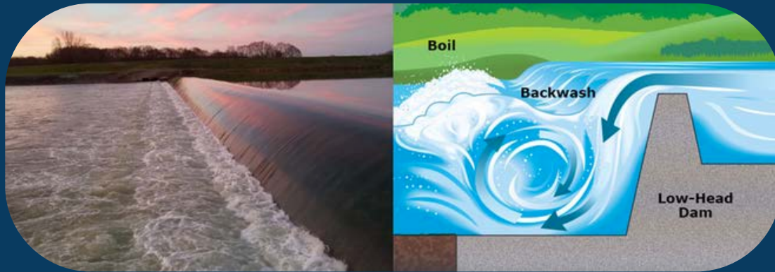
Image 1: A Low-head dam and illustration showing the backwash hydraulic affect that drowns unsuspecting swimmers and boaters. Photos: Public Domain
