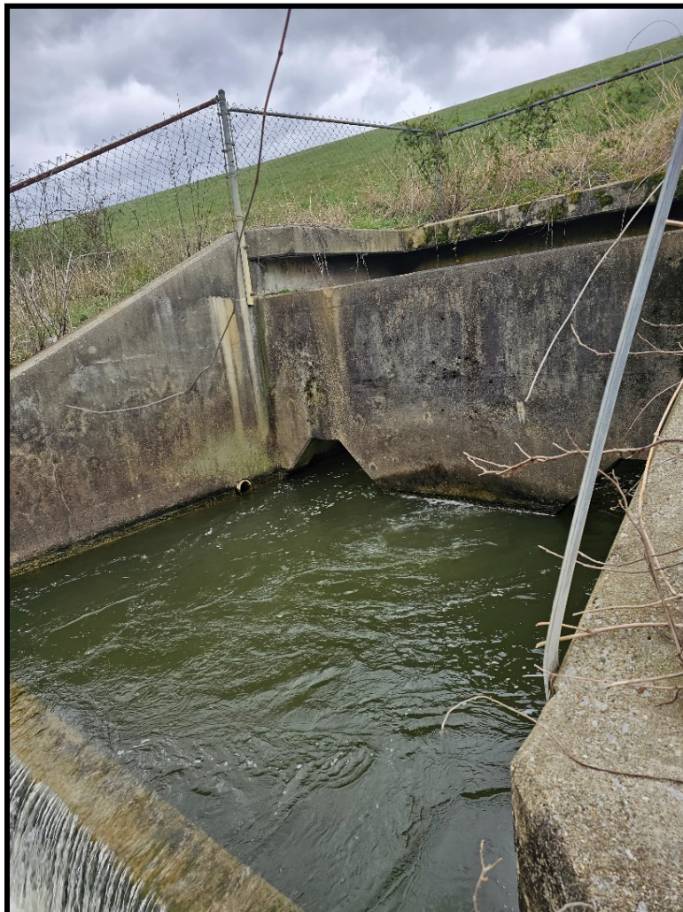
Figure 20. McDougal Lake Outlet Structure
