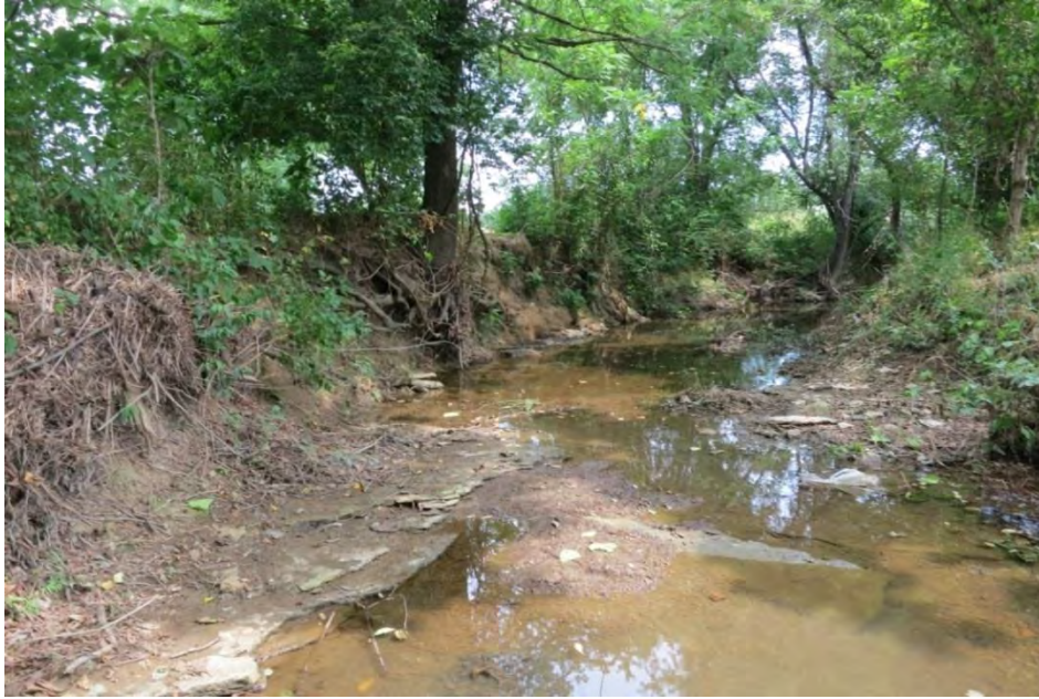
Figure 2.19: Stretch of Swift Camp Creek with eroded and incised banks (photo by Jon Walker 2012).
