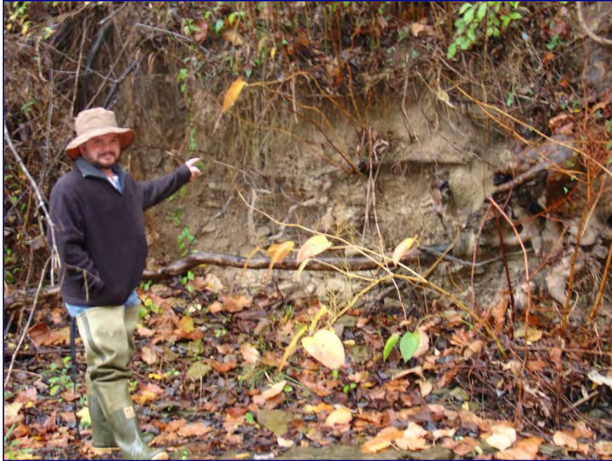
Figure 2.14 Photo showing erosion and mass wasting at a site on Dry Creek.
