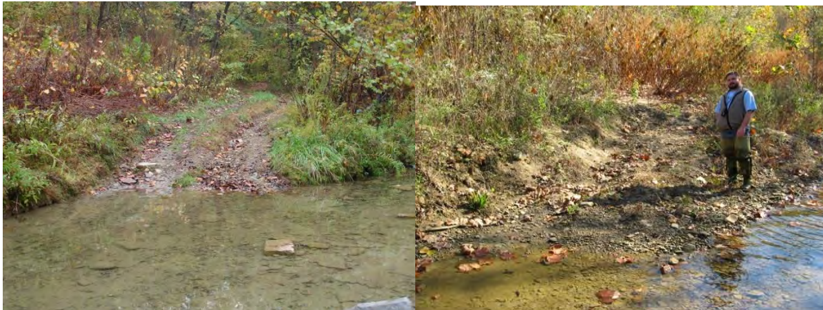
Figure 3.18: More unimproved access roads to Dry Creek streambed. Note fine-grained sediment deposited on the channel bottom, an example of impairment due to sedimentation/siltation. Most of the gravel has been removed in both images.
