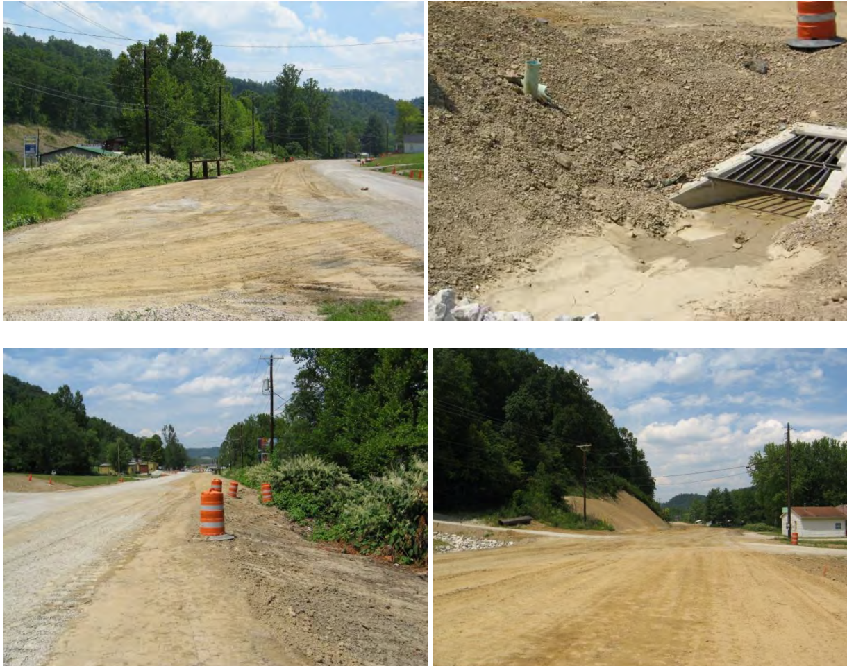
Figure 3.14: Sample of images taken during KY 519 construction, which show a complete absence of the erosion prevention and sediment controls required by state contracts.
