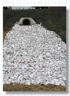
outlet pipe and the receiving stream is sufficiently wide to accept the divergence of flow, it is classed as a minimum tailwater condition.
