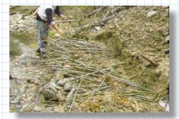
reinforce slopes by serving as tensile inclusions that provide frictional resistance to sliding or other types of displacement. The protruding brush retards runoff and reduces surface erosion.
