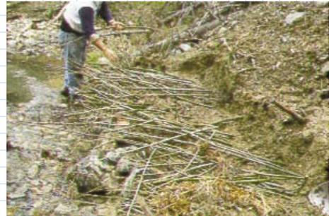
Brushlayering performs several functions for erosion control, earth reinforcement and slope stability:
