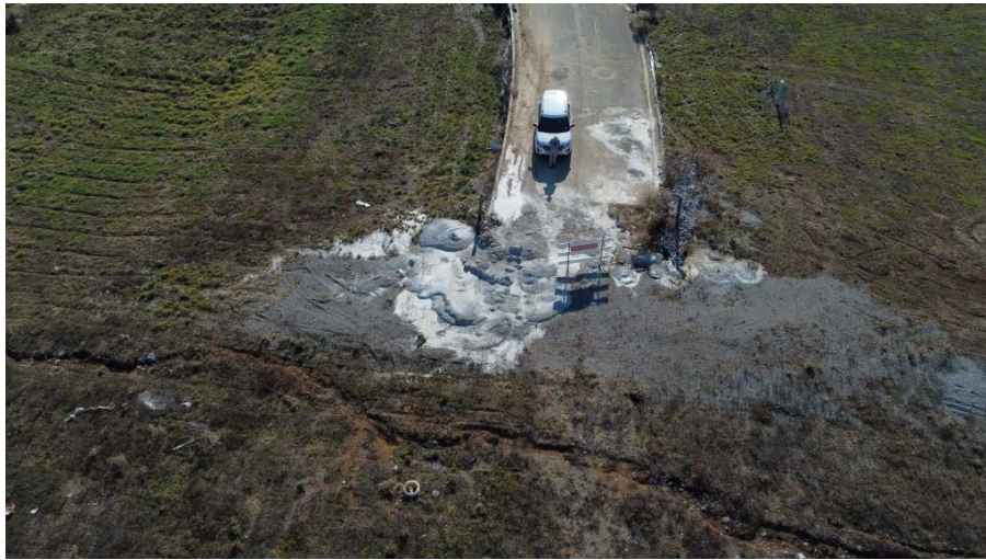
Improper concrete disposal
