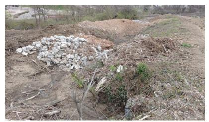
Poorly shaped rock check dam with mulch piled between the dams.
