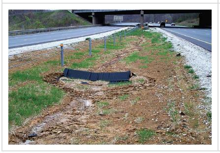
Poor application of commercial silt check product. Silt check needs to be longer (tied into banks). More are needed, at correct spacing for channel slope. Area needs to be reseeded; ditch may need blanket liner.
