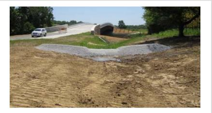
Good shaping of silt check dam. Note overflow at the top and width sufficient to cover all of ditch.
