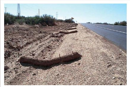
Good placement and spacing of fiber-roll silt checks. Coconut fiber rolls and other commercial products can be used where ditch slopes do not exceed three percent.
