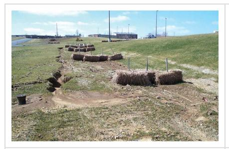
Poor silt check dam installation. Straw bales are not approved as silt checks for ditch or channel applications due to rotting, installation difficulties, and high failure potential.
