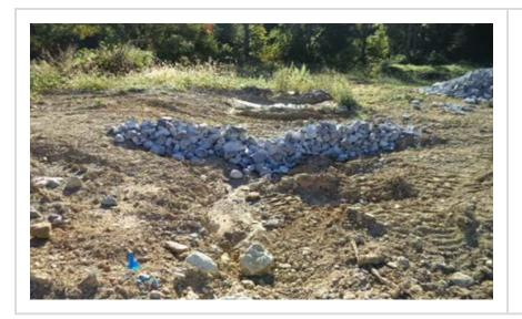
Aggregate too large and not appropriate width for channel. Channel poorly defined.
