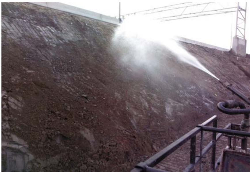
Treatment of a slope with polyacrylamide spray
