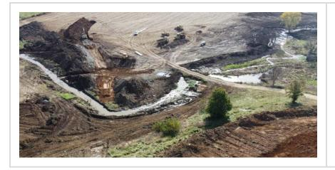
No protection for the stream at all. Equipment has been in the stream and not using the stream crossing. No erosion prevention on the site.
