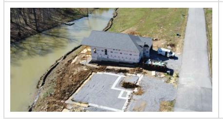
Good placement of silt fence, but it has failed and should be repaired to protect the stream channel. The gradient of this site would benefit from wattle or coir.
