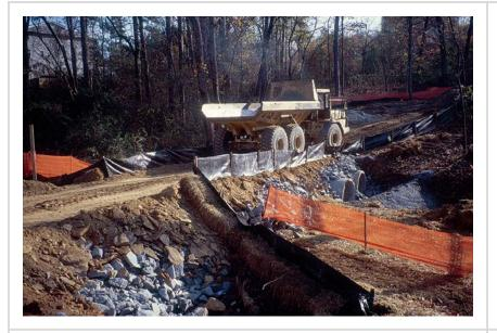
Good use of silt fence, straw, rock, and other practices for temporary stream crossing. Any work in stream channels—such as installation of culverts—requires a Section 404 permit from the U.S. Army Corps of Engineers and a Section 401 Water Quality Certification from the KY Division of Water.
