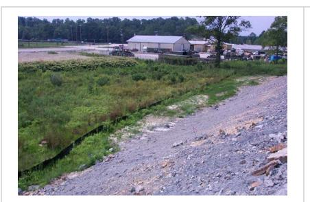
Use of silt fence to protect small intermittent stream adjacent to construction site. Note that native vegetation in the stream buffer area is not mowed, which promotes channel stability during high flows.
