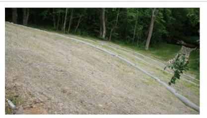
Good example of rolls along the slope with straw mat to aid in seeding and prevent slides. Rock channel on downhill side channeling flow to stream.
