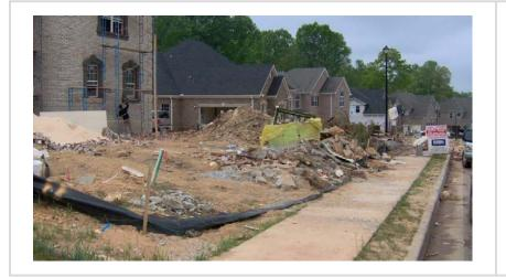
Poor solid waste, silt fencing, and other controls. Failure to control waste and sediment are violations of the KPDES Stormwater Permit.
