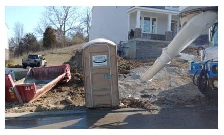
Poor sanitary facility placement. This is unlevel, in the path of traffic and on the edge of the culvert.
