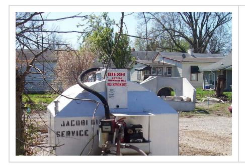
Double wall fuel tanks should be used. Locate them away from ditches, storm drains, and waterways.
