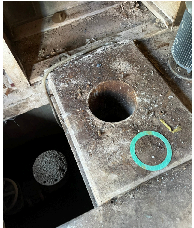
Figure 5. Warsaw Water Works, abandonment.
