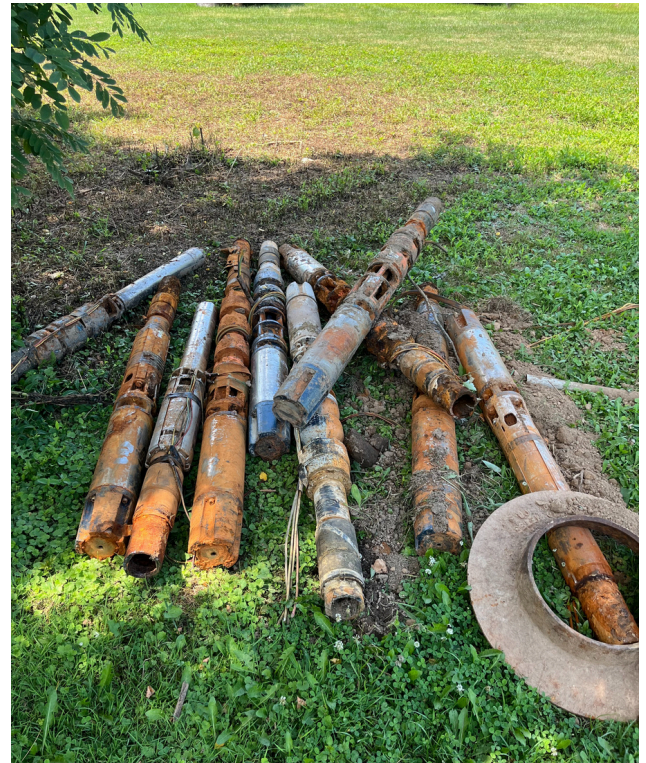
Figure 2. Well pumps removed from the abandoned wells at South Shore Water Works.
