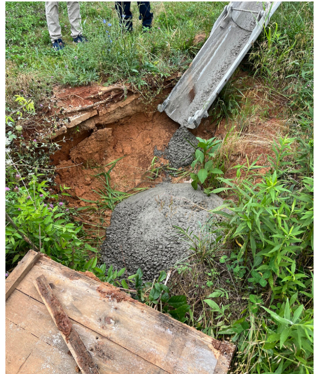
Figure 4. Hardin County #2, White Mills. Sealing the well shaft.
