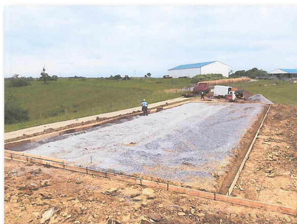
Construction of a heavy-use winter feed area to help reduce erosion from livestock-related physical disturbances.
