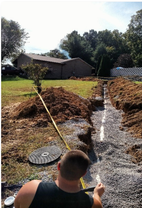
Connecting home to sewer system. Picture from: Lincoln County Homeowner Assistance Program Final Report.
