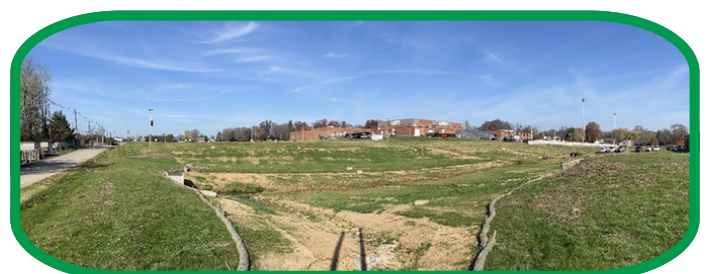
Figure 15. The completed stormwater bioretention basin along an upstream tributary of Lower Howards Creek.
