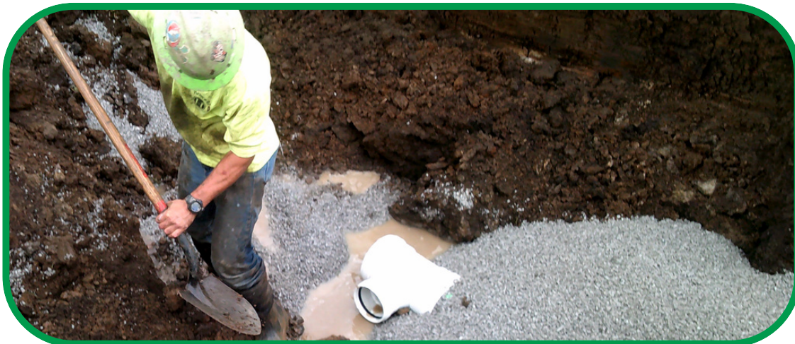
Figure 54 Workers in Scott County connect residents to new sanitary sewer
