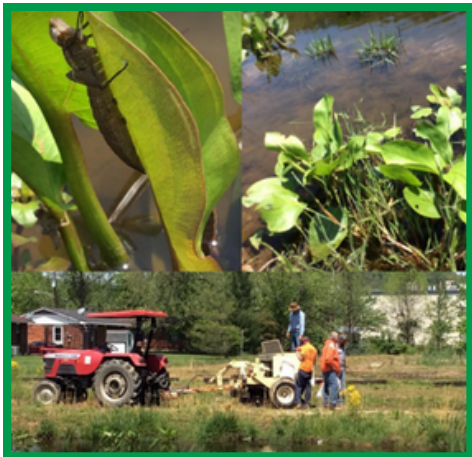
Figure 2. Green infrastructure Wetlands installed in the watershed.
