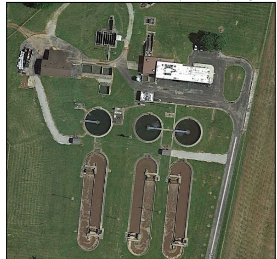
Princeton Wastewater Treatment Plant
