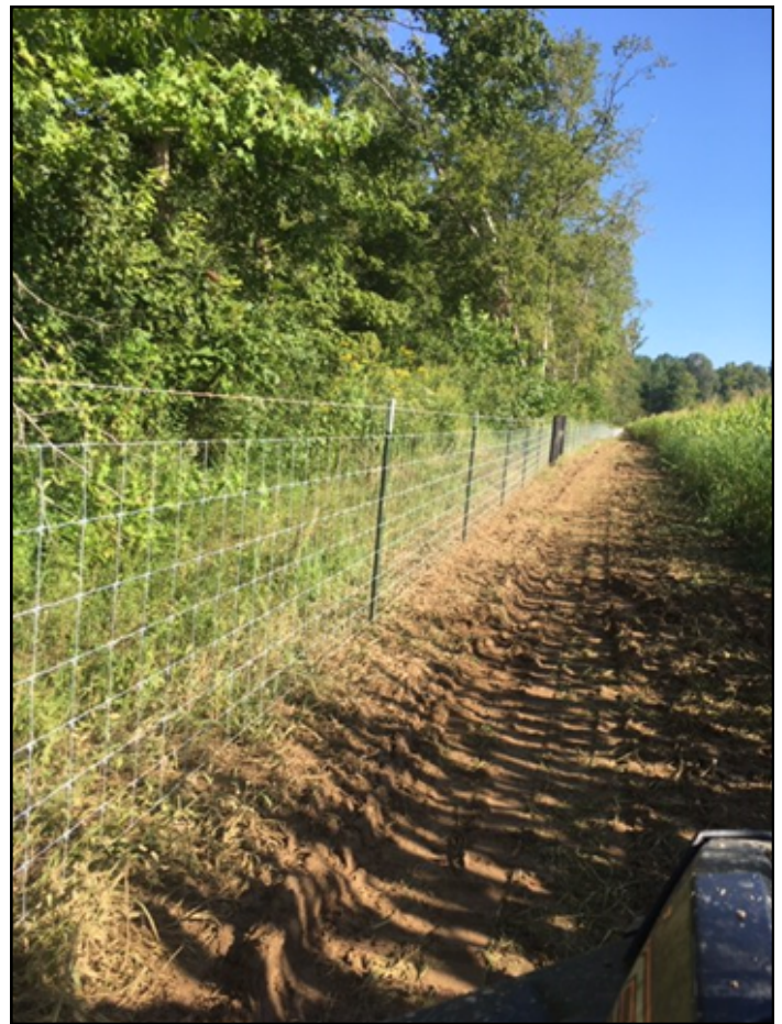
Figure 5. New Livestock exclusion fencing installed to protect a streambank and riparian buffer.
