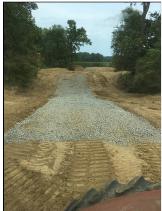
Figure 7. Hardened stream crossings installed to protect streambanks while accessing crop fields.
