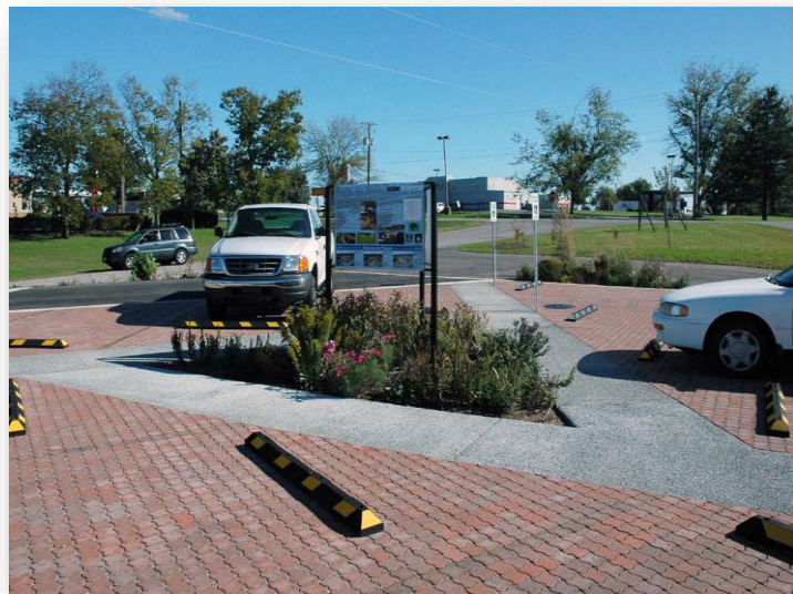
Figure 6.1. Pervious parking lot and rain garden at Georgetown, KY fire station.
