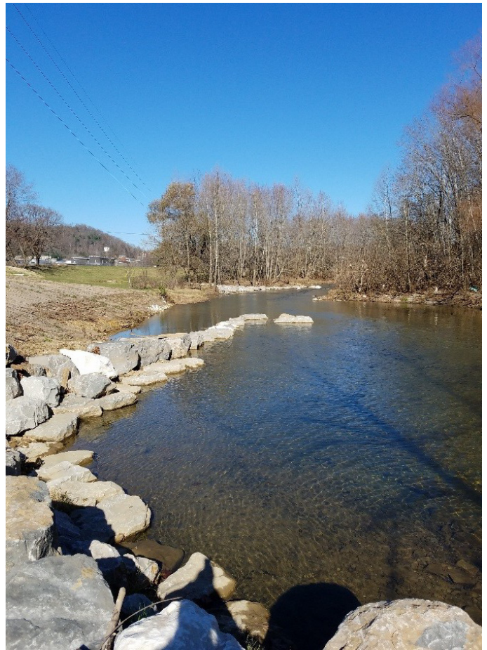
Triplett Creek stream stabilization site with J-hooks and sloped banks
