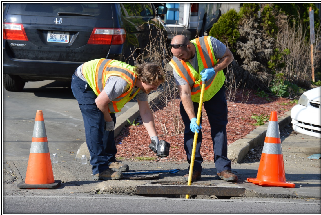
Figure 2.2.2: SD1 performing an IDDE inspection
