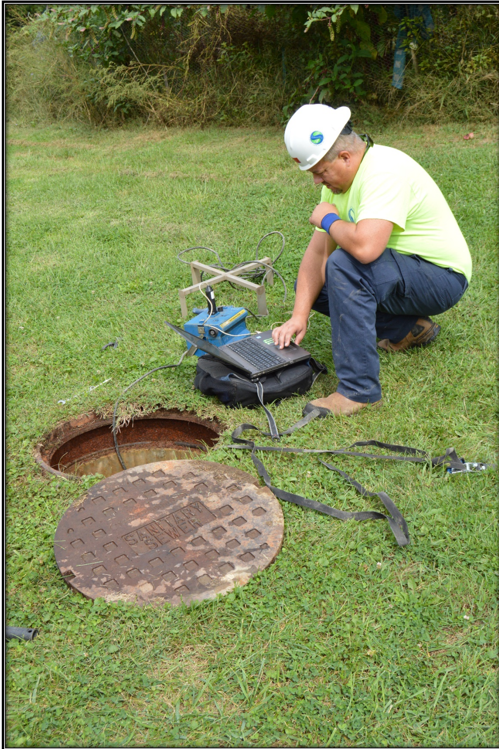
Figure 2.4.2: SD1 performing a sanitary structure inspection
