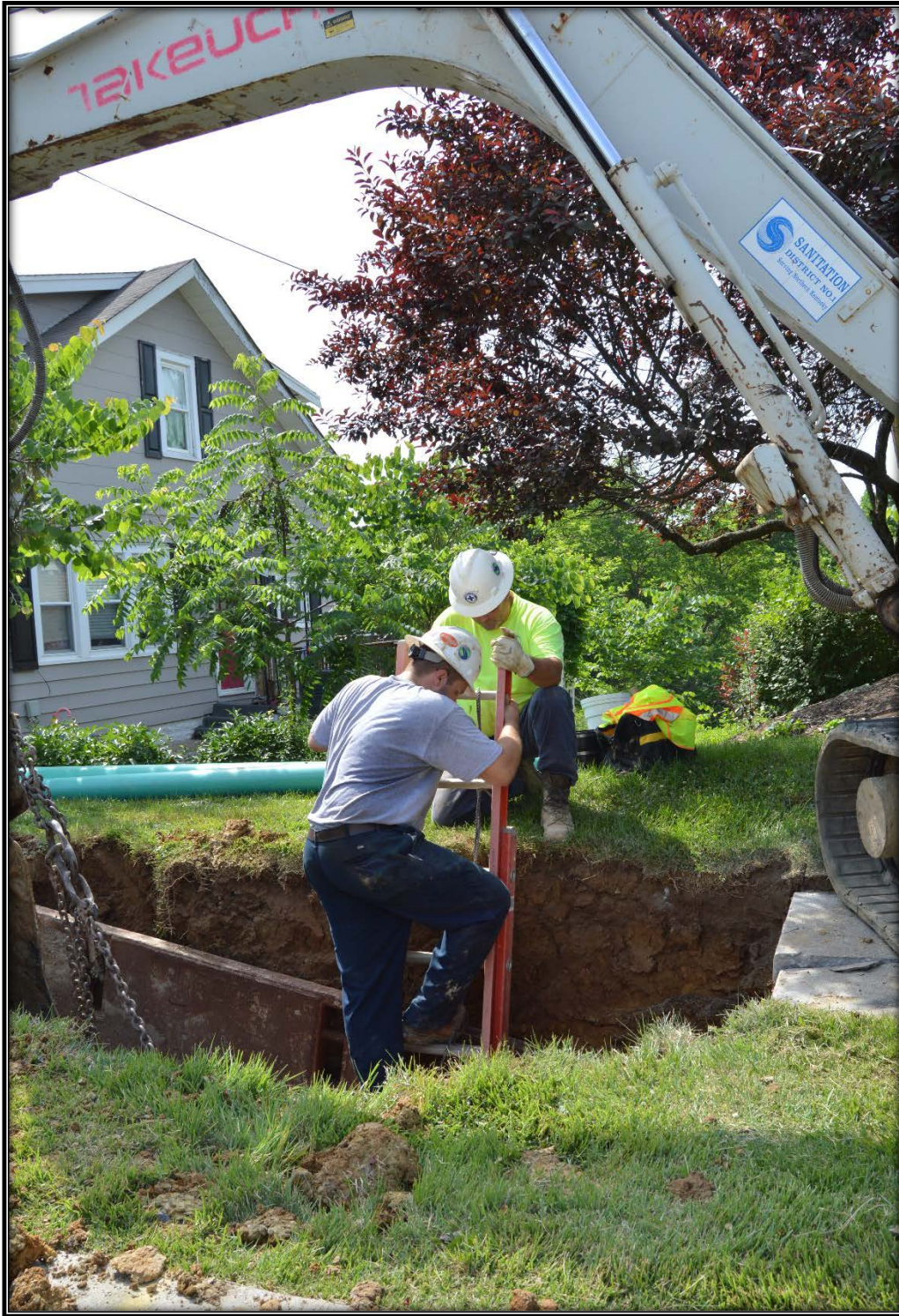
Figure 2.5.2: SD1 performing sewer maintenance and repair
