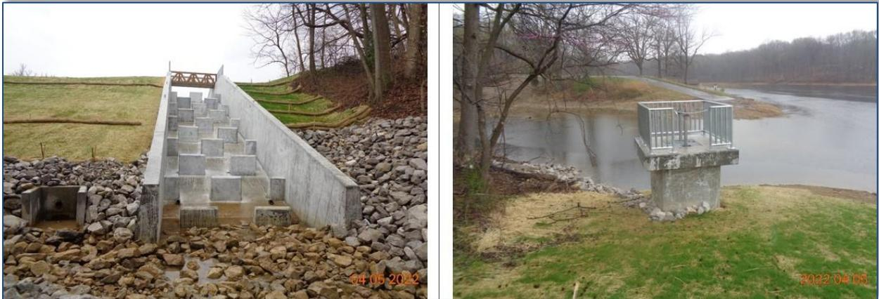
Scenic Lake Dam: new spillway and riprap stilling basin (L) and drawdown system tower (R)
