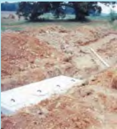
Septic system installation
