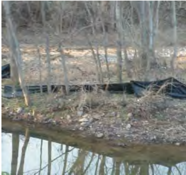
Silt fence at construction site
