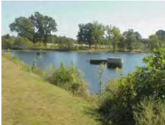
Drinking water intake structure
