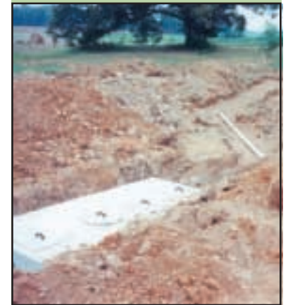
Septic system installation
