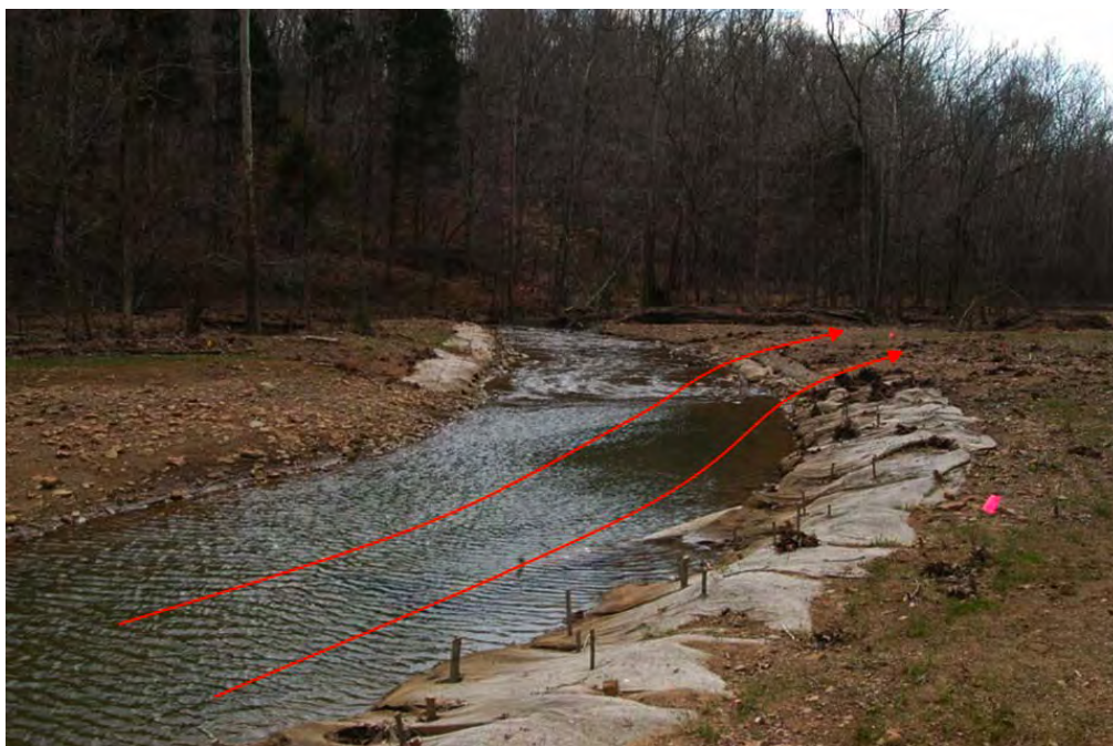
Figure 3 Flood flow overtops banks as it leaves the bend of the restored channel prior to sod placement. Note the erosion control matting is still in place at the toe of the bank downstream of the bend. Ruts have formed in the unvegetated floodplain and on the top of the bank near the flow indication arrows.
