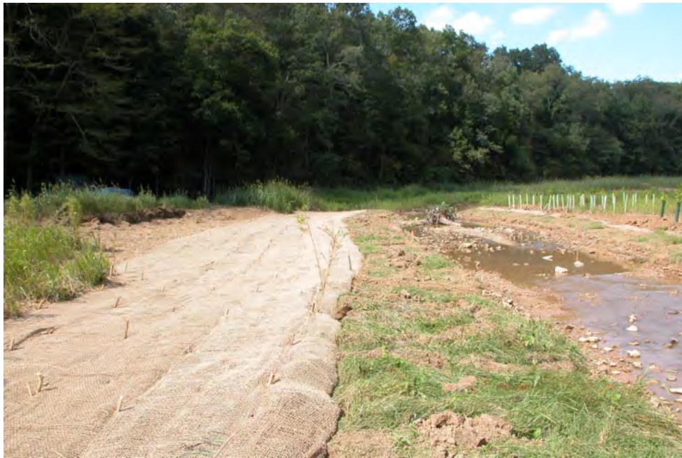
Figure 3 Sod mats adjacent to stream directly following installation. Erosion mesh is tied into the sod and covers much of the floodplain
