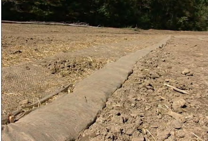
Figure 2: Newly constructed riffle in stream restoration before introduction of flow to the channel. Anti-Wash Geojute™, burlap wrap, and stream channel are pictured from left to right
