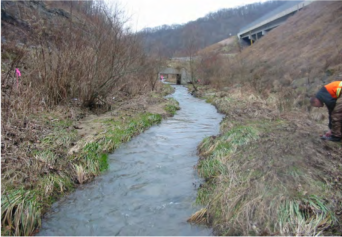
Figure 3.2 Stable, well-developed active floodplain within a constructed flood conveyance channel along Road Fork, Pike County.
