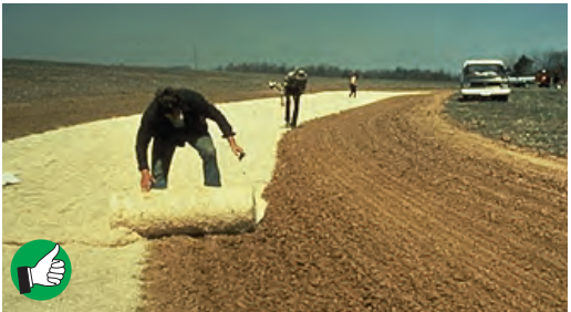
Blankets installed along stream banks or other short slopes can be laid horizontally. Install blankets vertically on longer slopes. Ensure 6 inch minimum overlap.
