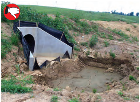
Poor seed and mulch application, slopes badly eroding. No rock apron or flow dissipater at culvert outlet. Culverts clogged with sediment and rock.
