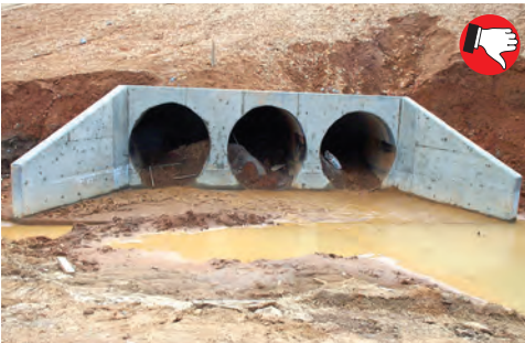
Poor seed and mulch application, slopes badly eroding. No rock apron or flow dissipater at culvert outlet. Culverts clogged with sediment and rock.
