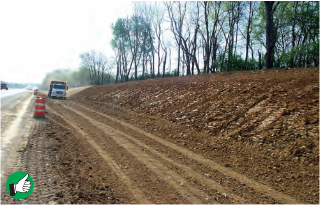
Excellent soil conditioning (dozer tracking) prior to seeding and straw-blowing. Seed and mulch provide cheap, excellent protection. Use blankets on slopes if they are steep or soils are poor.
