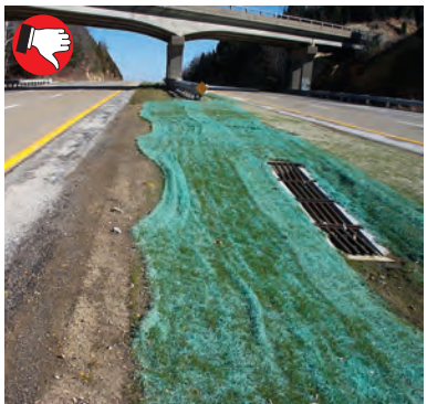
Good application of erosion control blanket to stabilize shoulder and protect storm drain, but too few staples used along the top edge. Trench in top edge of blanket on steep slopes.
