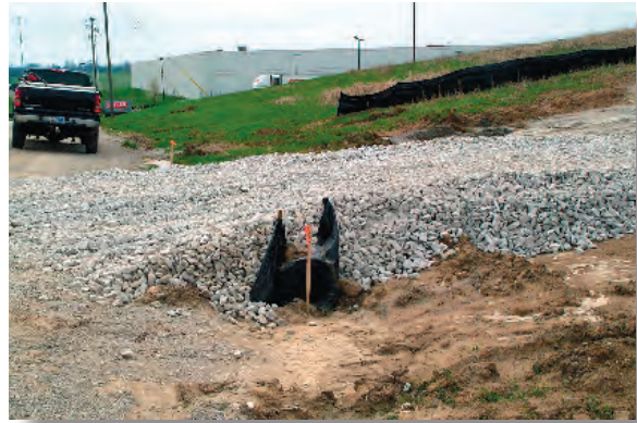
A well-maintained construction exit keeps mud off the pavement and helps to reduce potential legal liability.
