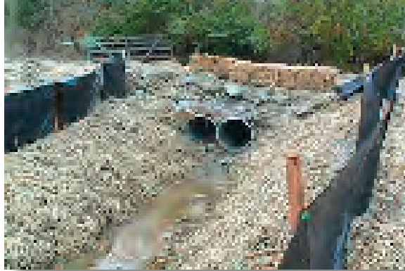
Temporary stream crossings require a USACE Clean Water Act section 404 permit. Avoid or minimize removal of vegetation and excavation at the crossing site. Cover all bare soil areas with straw or ECBs. Cover the approaches on both sides (25 ft minimum) with No. 2 stone.
