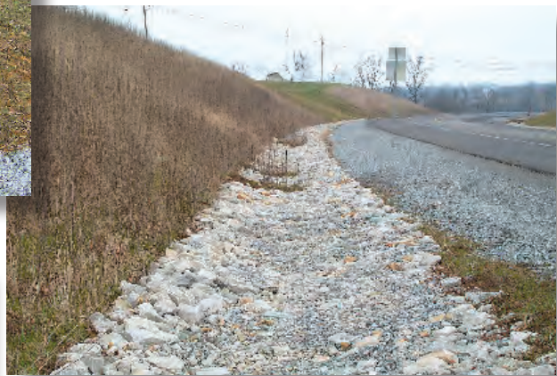
This shows a very good stabilization of slope and ditch on highway project. Note the mix of large and small rock, which helps fills voids and deters undermining.
