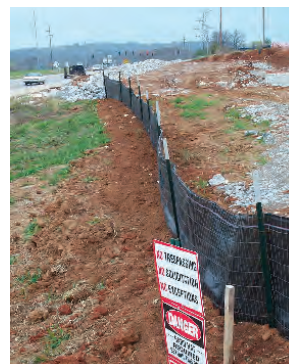
Super (wire reinforced) silt fence in the foreground, supplemented by rock sediment barrier (background). Use rock or other sediment barriers when appropriate.
