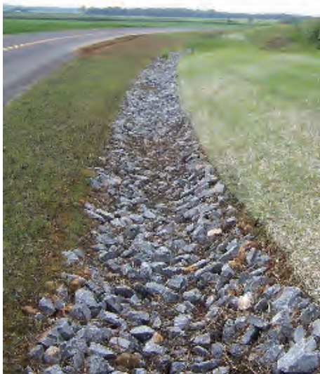
The rock is a little thin along this ditch, but could be acceptable because of the lack of visible channel erosion. Ditches should be monitored so that rock or other protective controls can be added if erosion becomes a problem.
