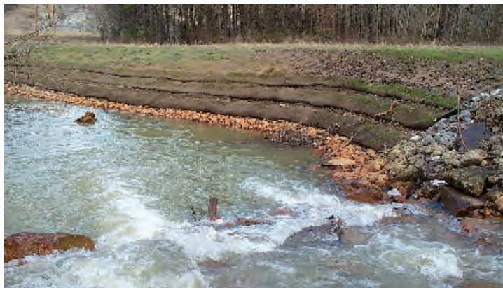
Soil wrap stabilization of steep stream bank using geotextile wrapping in 2 ft lifts. Live stakes can be driven into prepared banks using a dibble bar or iron stake to create a guide hole.
