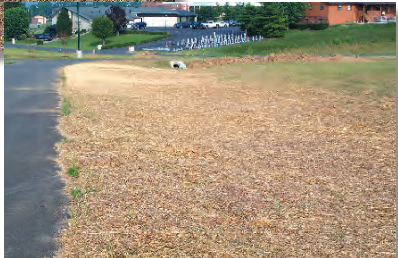
Good use of straw mulch and grass seed in relatively flat and fairly wide swale. For more concentrated flows, triple seed the ditch and use erosion control blankets.
