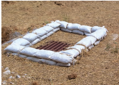
Inlet protection berm constructed of half-filled stone bags. Use #57 rock, overlap bags to eliminate large openings and rapid flow-through. Construction-grade bags of netting material—similar to onion bags—can also be used.
