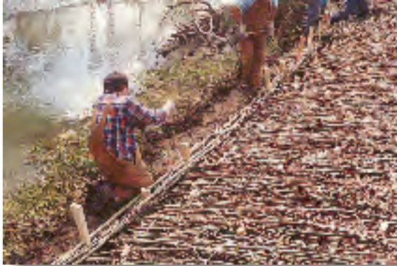
Installation of live fascines along bank area, before backfilling. Fascines provide quick, thick growth to stabilize banks and can be specified where willow or other suitable plant material is plentiful and erosive forces are moderate. Use turf reinforcement mats in areas where bank shear stress exceeds 2 pounds per square foot.
