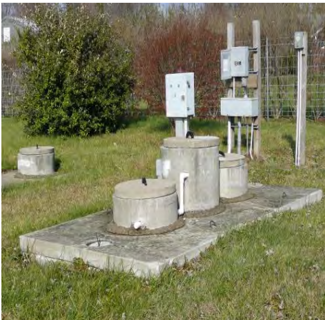
Figure 3. Gribbins Whirlair Aeration Unit
