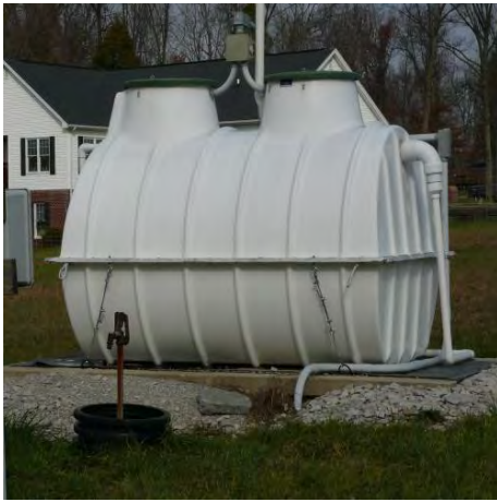
Figure 8. Chromoglass Batch Reactor
