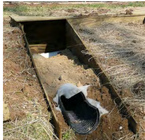
Figure 17. Gravelless Pipe Display
