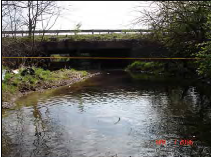
Clarks Run Bypass - Non-select site at the Danville US127 Bypass for characterizing potential nutrient and bacterial contribution from industrial and some residential sources. Located at 37.627177, -84.797265.
