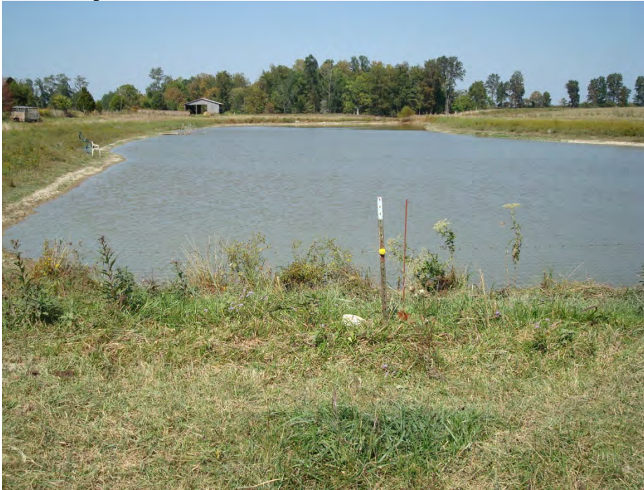
Pond Ramp: Before
