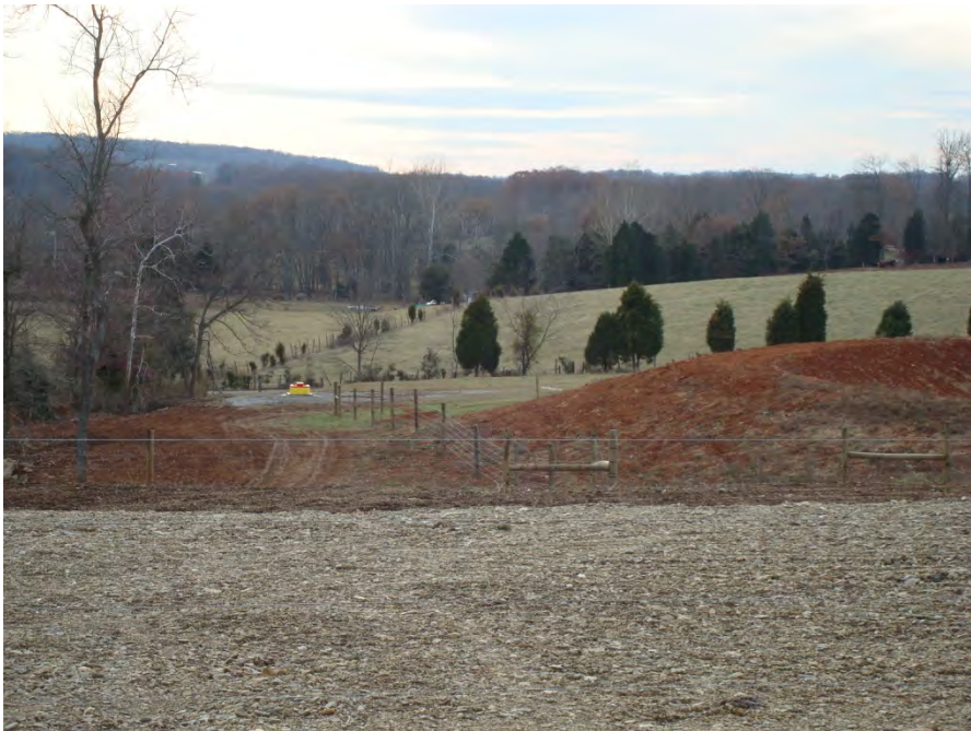
Pond Tank: After
