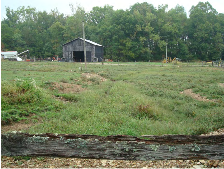
Stream Crossing: Before
