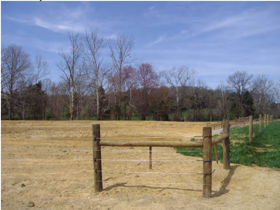
Pond Ramp and Fence: After
