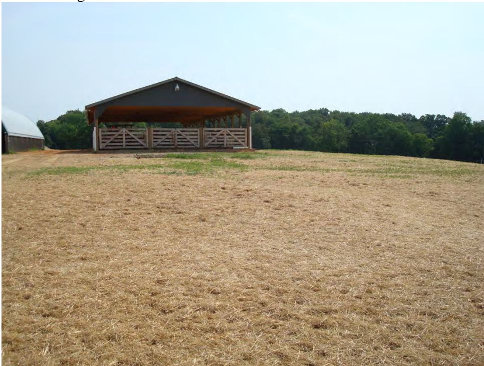
Waste Storage: After
