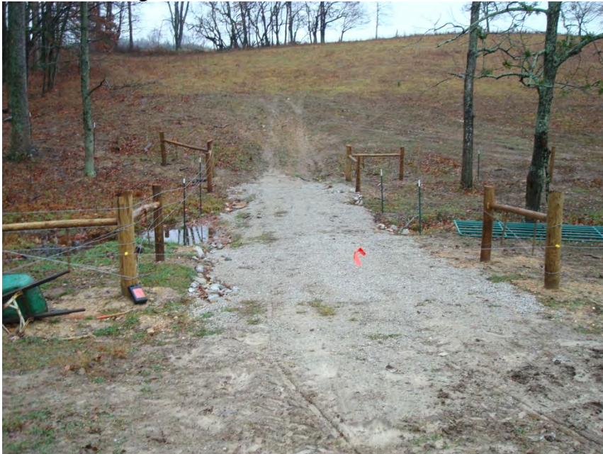
Stream Crossing: After
