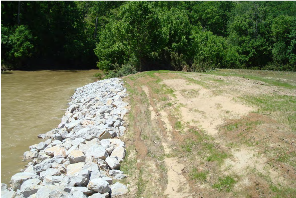
Streambank Protection: After
