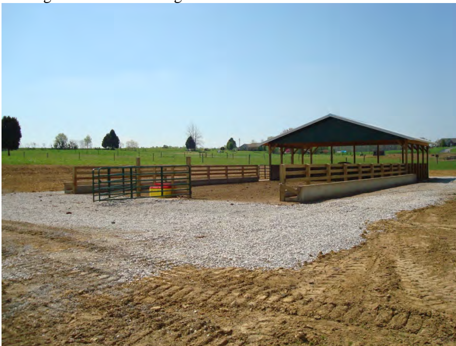
Feeding Area/ Waste Storage: After
