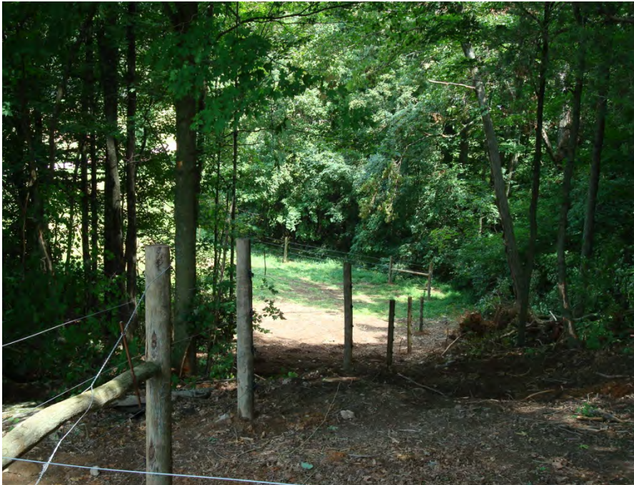
Woodland Fence: After
