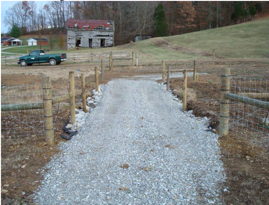
Stream Crossing: After
