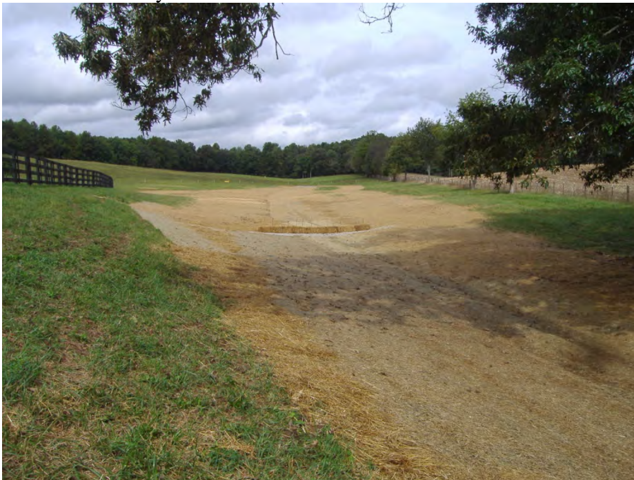
Grassed Waterway: After
