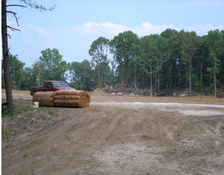
Figure 10: Impoundment after backfilling, limestone barrier application, and suitable cover material placement.
