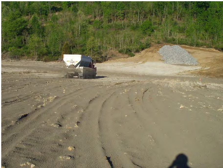
Figure 9: Agriculture Limestone barrier application
