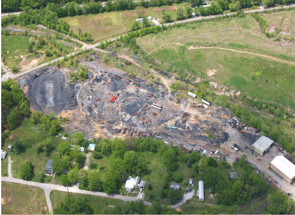
Figure 7: Nortonville Refuse Area.
