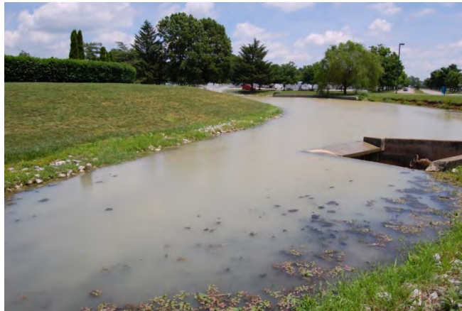
Figure 32. Sand runoff and deposition in this pond resulted in shallow water depth, higher water temperatures, and algae blooms .
