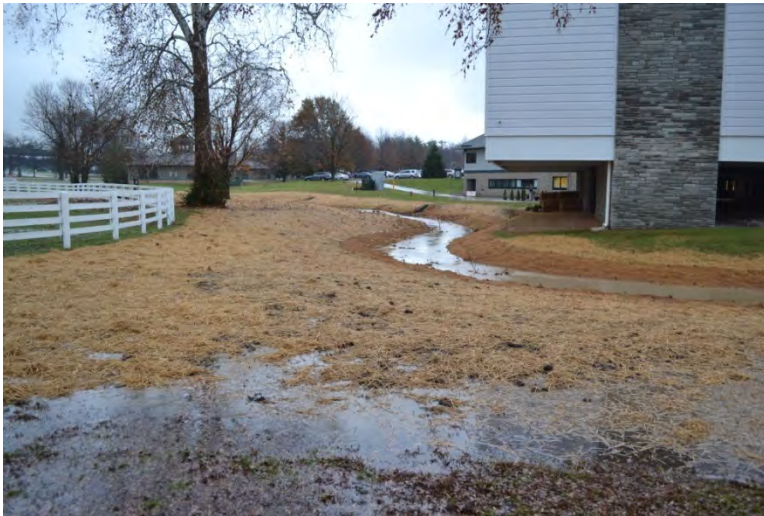
Figure 41. A floodplain was created to allow excess water from large rain events to escape from the stream channel, thus limiting streambank erosion
