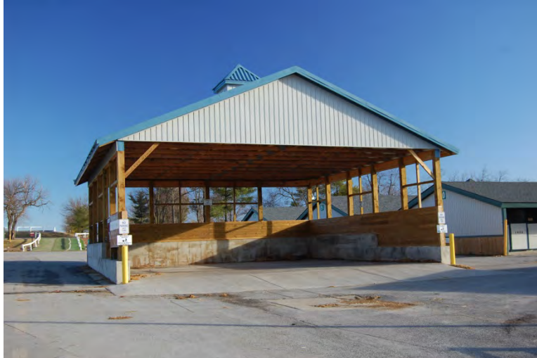
Figure 44. A waste storage facility was constructed to provide a designated, covered storage area
