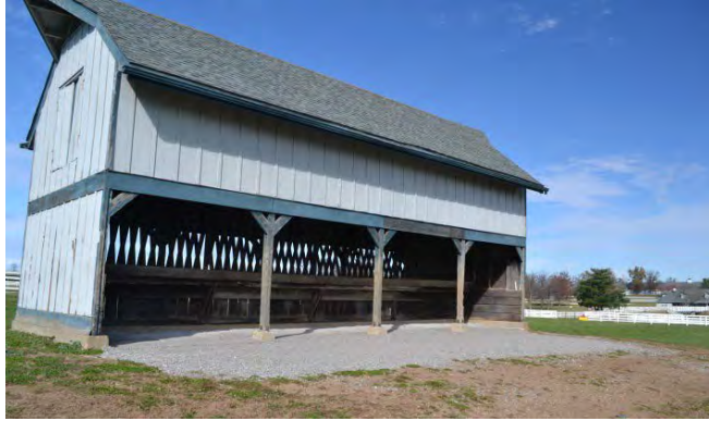
Figure 26. One of two HUAs installed outside of a run-in shed
