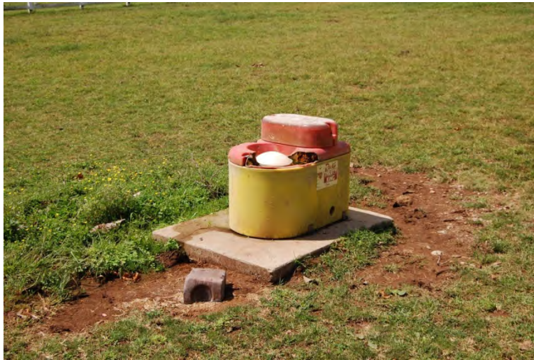
Figure 21. A dilapidated watering fountain that was poorly sited and not placed on a proper HUA
