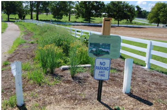
Figure 24. A bioswale and educational signage installed in a stormwater ditch.
