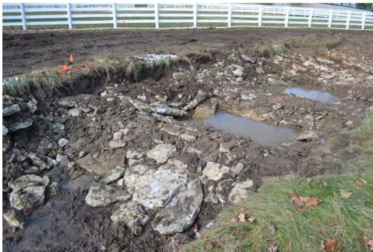
Figure 43. Pools and riffles were created to slow velocity and create habitat for macroinvertebrates and other aquatic life
