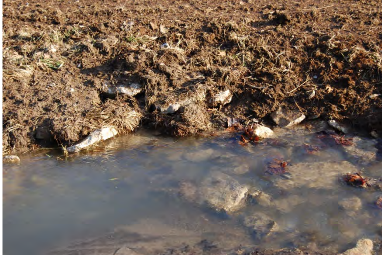
Figure 42. Stream banks were stabilized with toe rock in various sections
