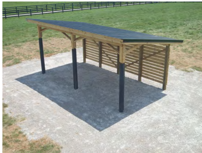
Figure 16. Heavy use areas were installed under 4 permanent shade structures with UK CAFE funds
