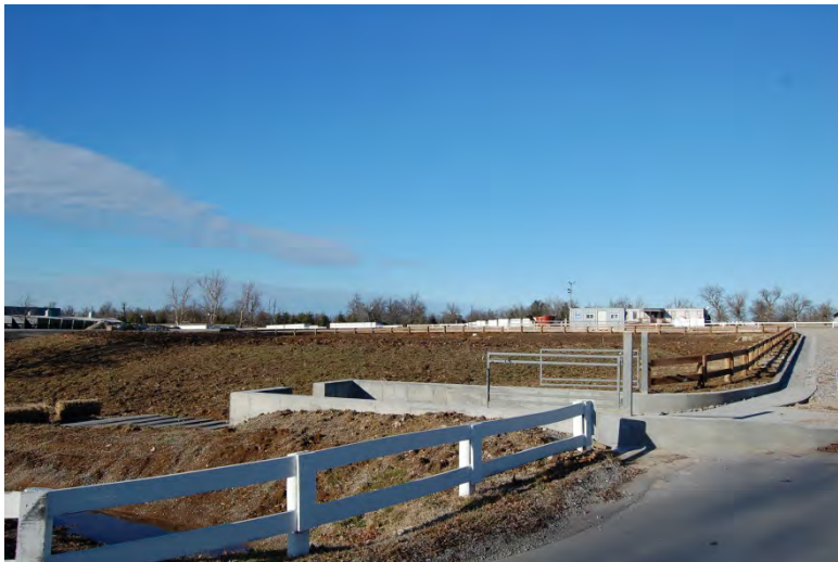
Figure 36. A settling basin was installed in a gravel parking lot at the KHP and labeled with educational signage
