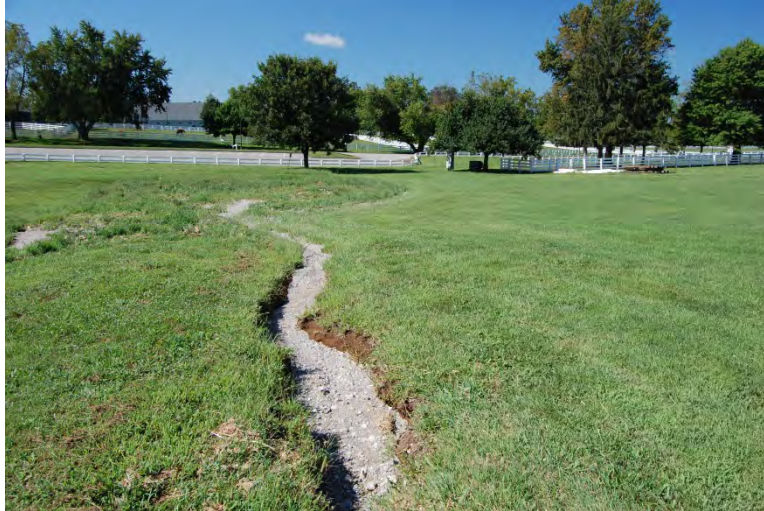
Figure 37. Prior to the settling basin's installation, runoff from the parking lot was carrying gravel offsite into the stream channel
