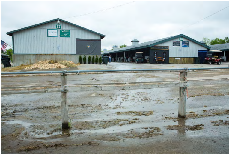
Figure 45. Prior to building the waste storage structure, manure was piled at the end of barns, uncovered
