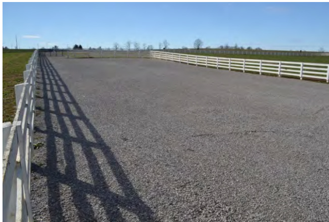
Figure 27. Large HUA installed in trail horse paddock
