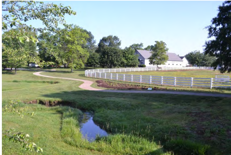
Figure 33. A rain garden was installed to filter runoff from the uphill, partially denuded paddock
