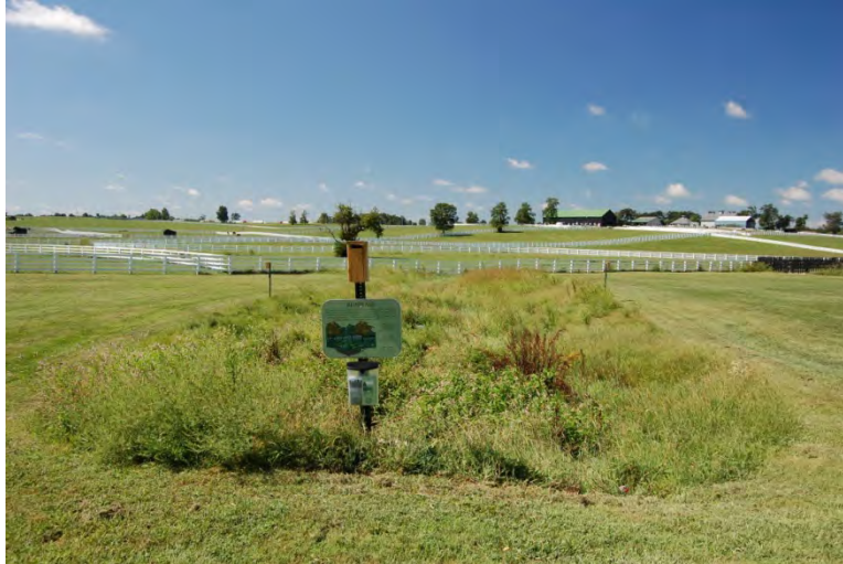
Figure 25. A bioswale and educational signage installed in a stormwater ditch.
