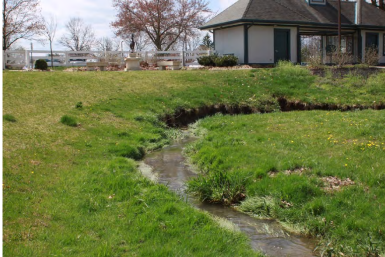
Figure 40. A section of an unnamed tributary lacked floodplain access and concentrated flow resulted in gulley formation.
