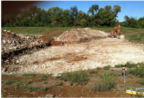
Fig. 8: Constructing bio-infiltration basin
