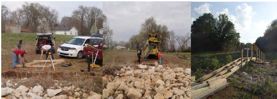
Fig. 33 Campus Habitat for Humanity students work on constructing pedestrian bridge
