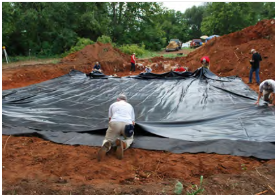
Fig. 27: Volunteers lay the pond liner
