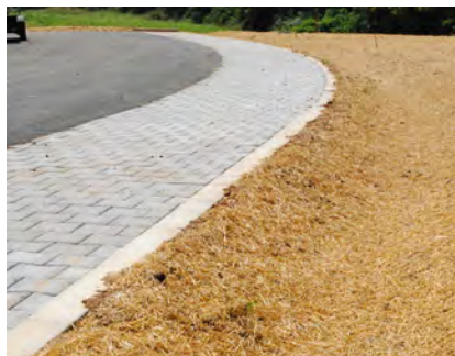
Fig. 11: Permeable pavers parking lane
