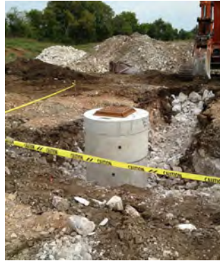
Fig. 9: New injection well with French drain
