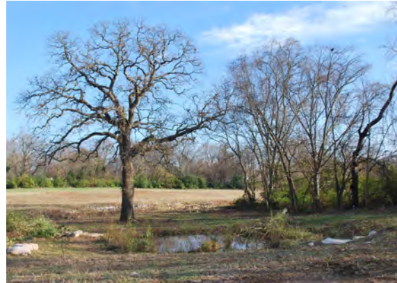
Fig. 28: Completed vernal pond in late fall-winter
