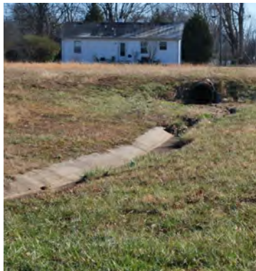
Fig. 5 Concrete drainage channel
