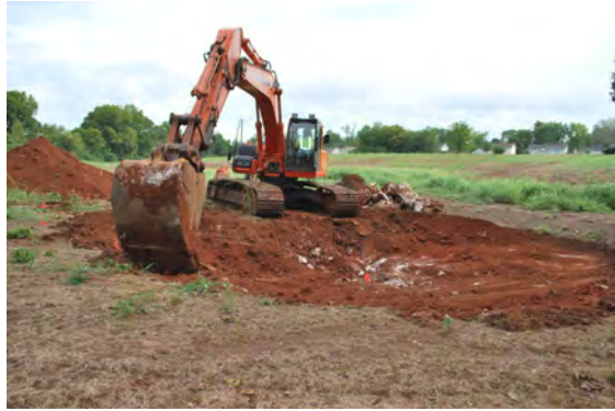
Fig. 26: Heavy equipment digs for vernal pond
