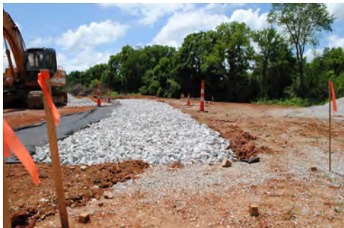
Fig. 10: Preparation for permeable pavers
