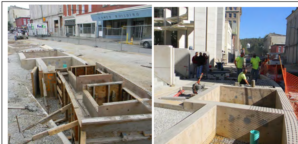
Figure 9 – St. Clair St. Rain Garden – under construction (CDP)
