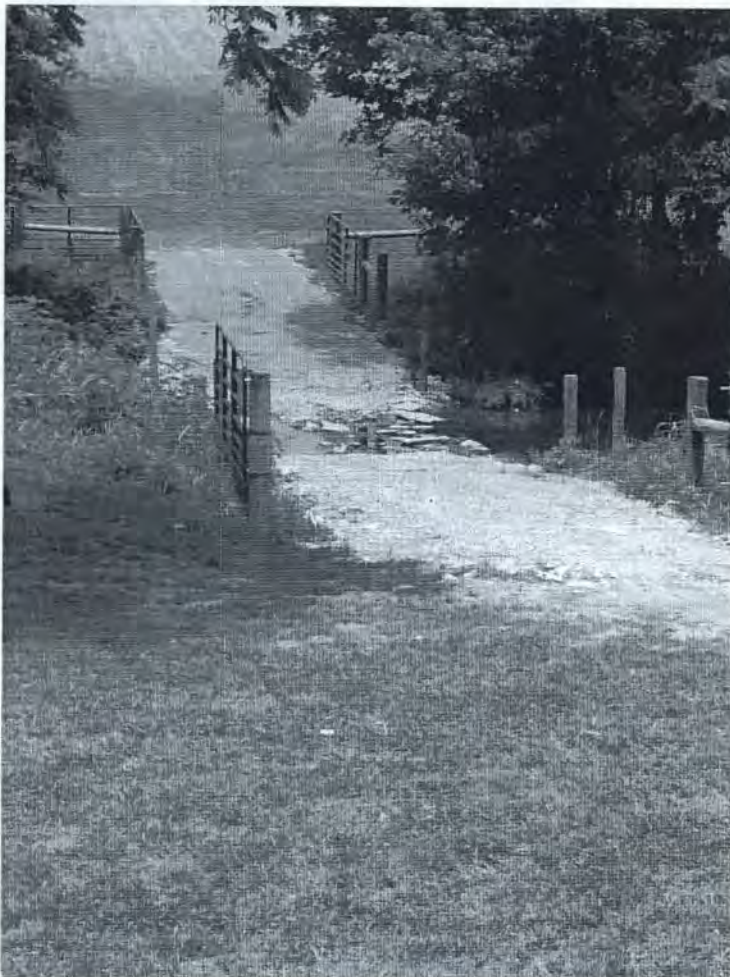
Stabilized livestock stream crossing and stream exclusion fencing installed via project cost share funding at the Erin Perdue farm in Bourbon County, Kentucky.
