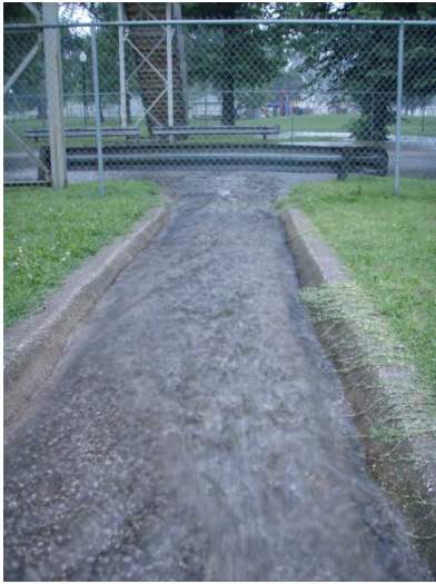
Image B - Flume before modification, flow to street.
