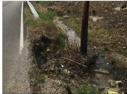
(Left) Metal posts have been inserted to address roadway washout associated with erosion on Sandlick Creek near Dan's Crossing Road. (Right) Roadway washout along Dry Fork near Heartbreak Ridge due to erosion.
