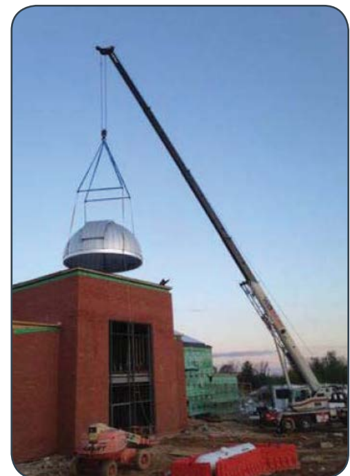
Dome being placed on top of the new APUS Information Technology Center
